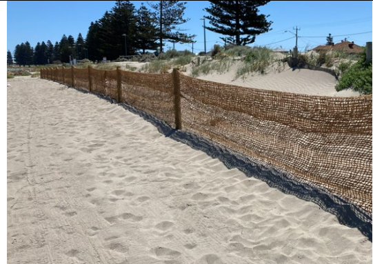
Sand drift impacting pedestrian path and new preventative fencing installed – Safety Bay Foreshore
