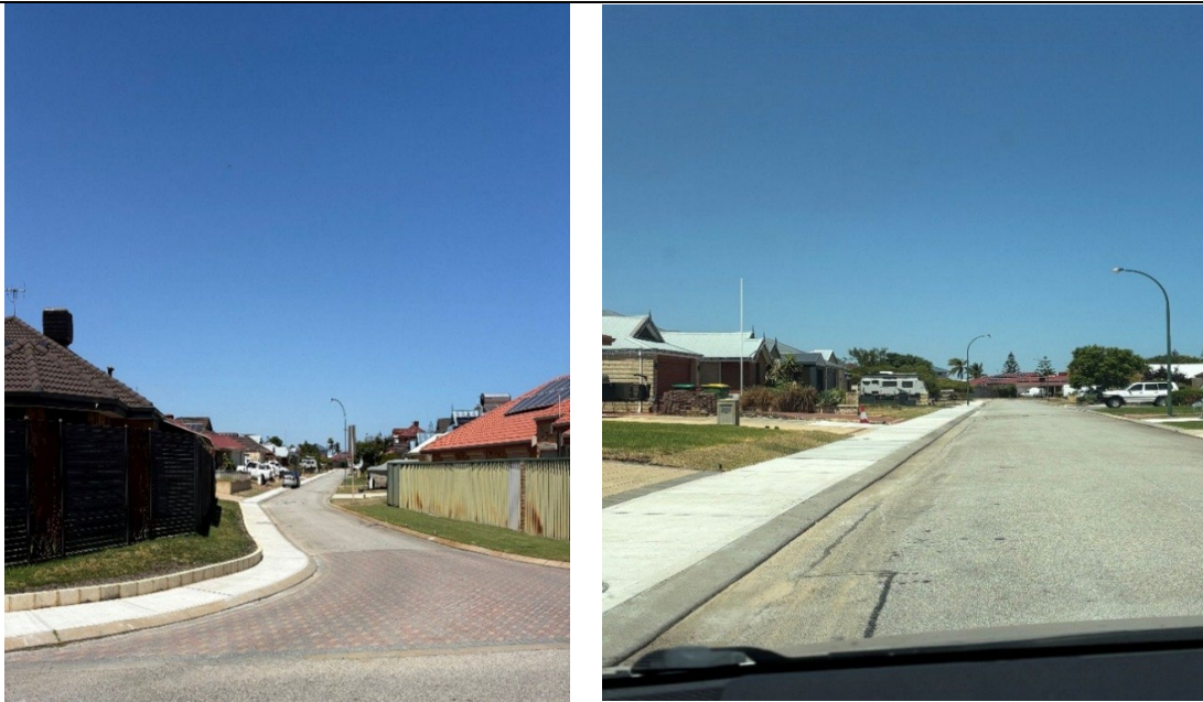
Completed footpath – Bluefields Parkway
