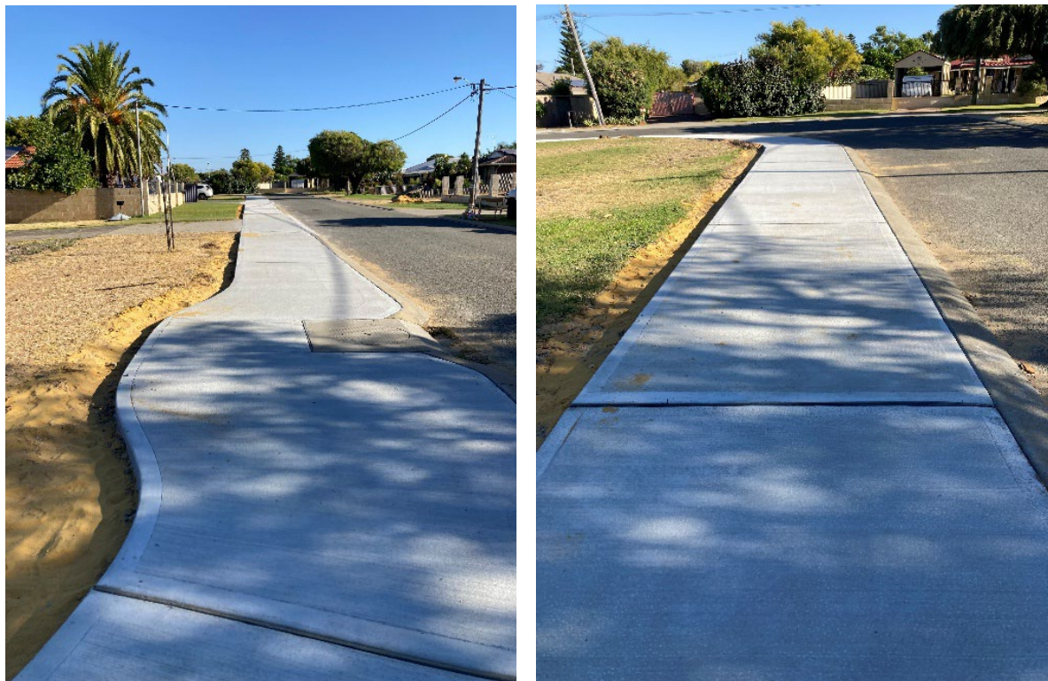
Works in progress
