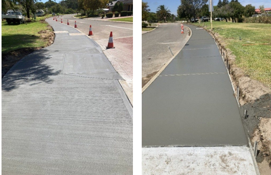
Works in progress
