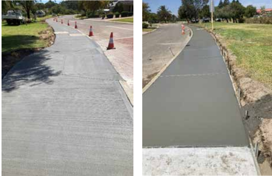
Works in progress
