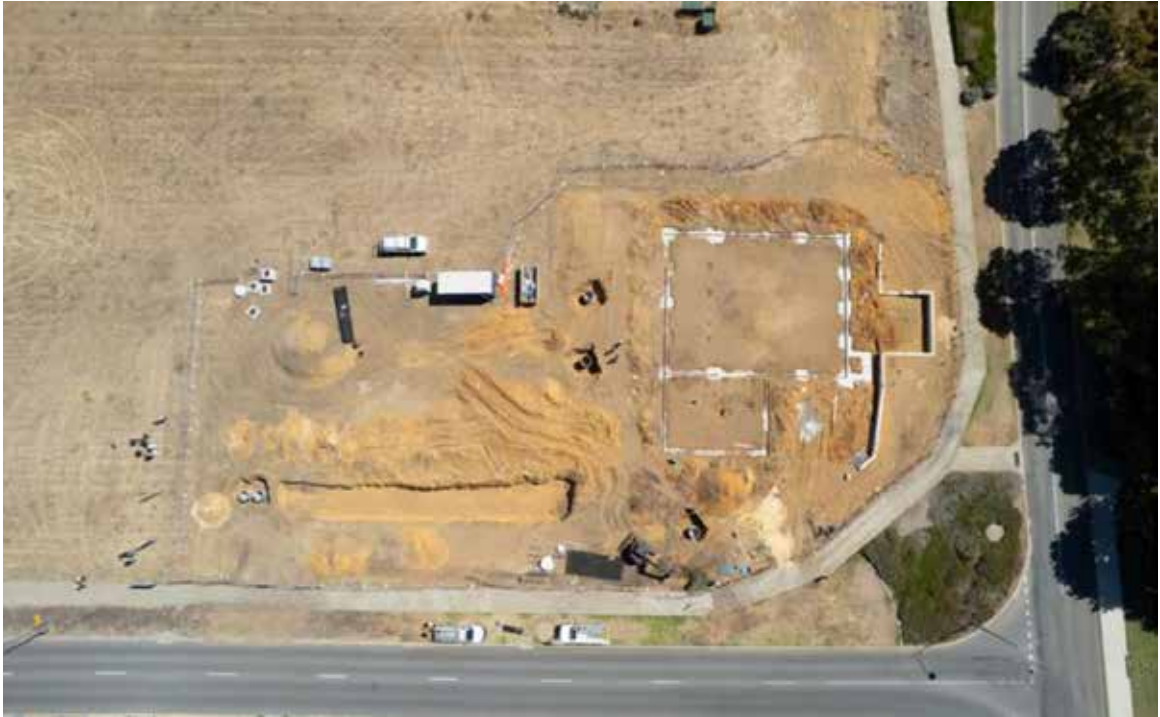
Photo 1: Baldvis Men's Shed – Aerial View of Site
