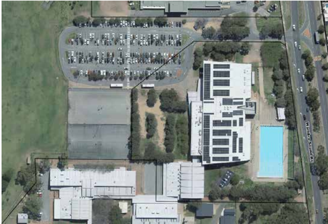
1. Aqua Jetty current aerial photo
