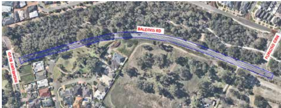
Section of Baldvis Road
