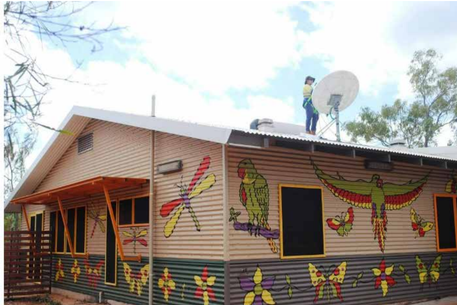
Image of Satellite Equipment Installed at Mike Barnett Sports Complex
