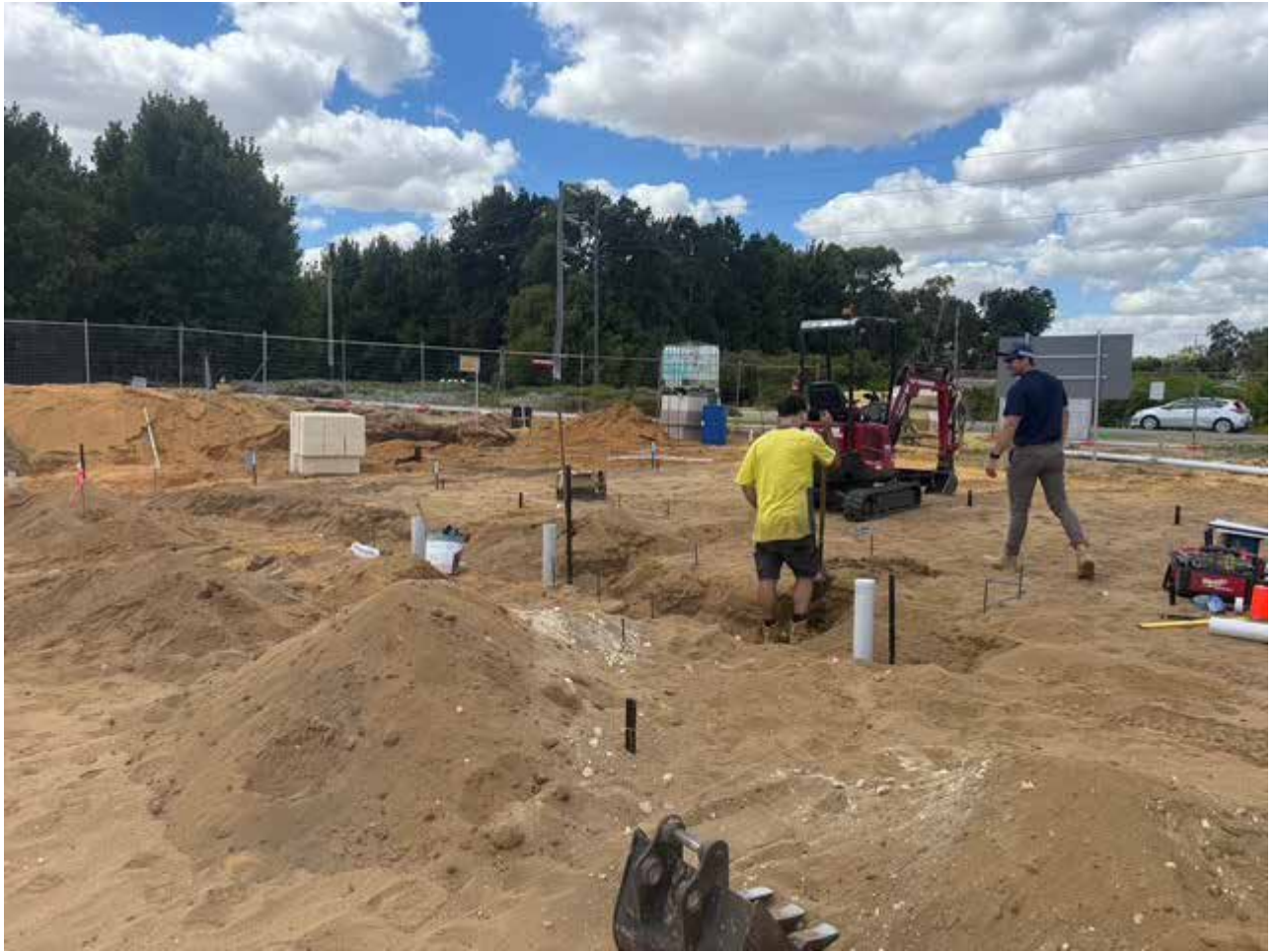
Photo 1: Baldvis Men's Shed – Installation of plumbing services
