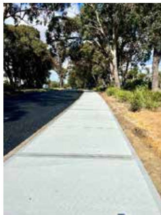
Works in Progress
