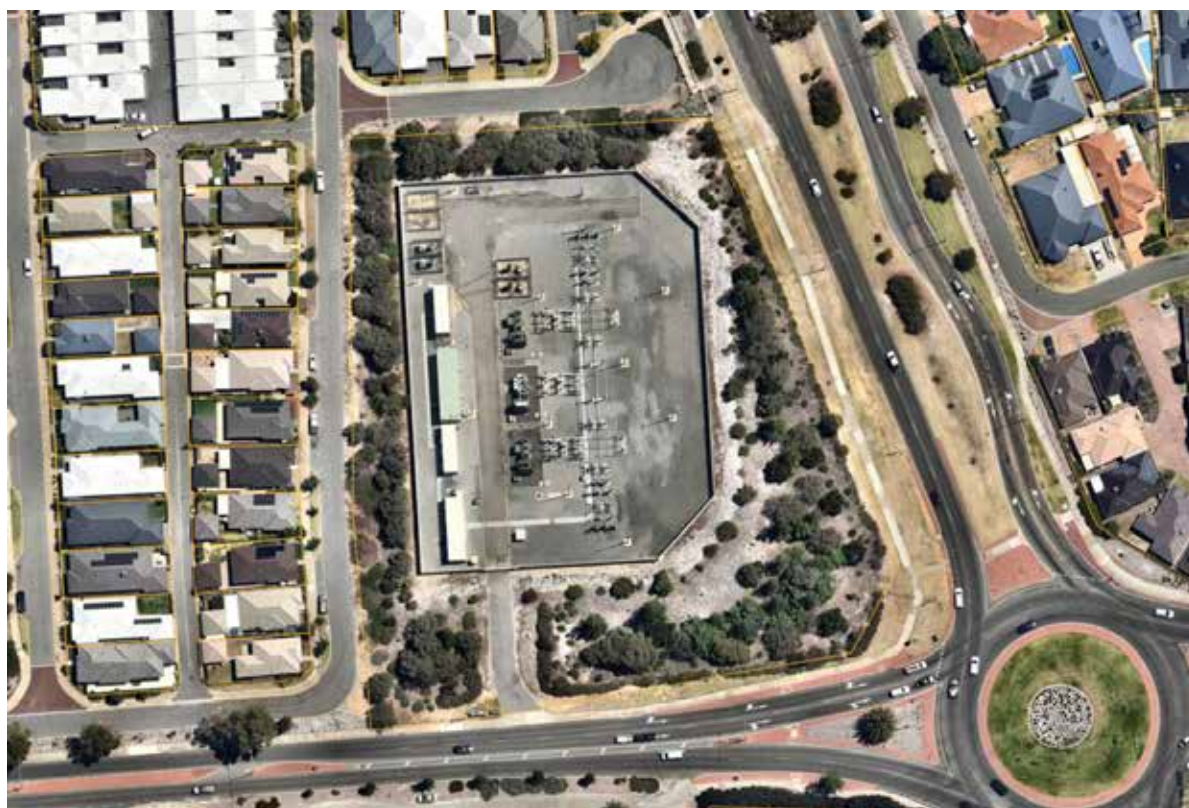
2. Existing Waikiki Zone Substation (WAI)
