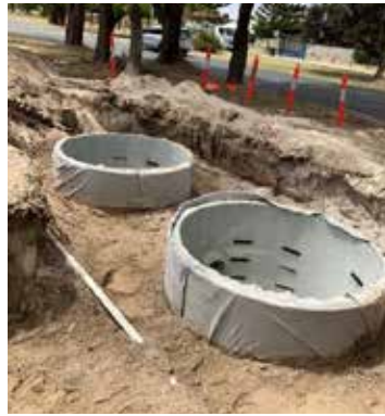
Read Street works in progress
