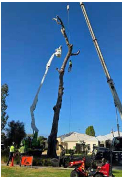
Crane and Elevated Work Platform commencing tree removal, Province Reserve, Baldivis
