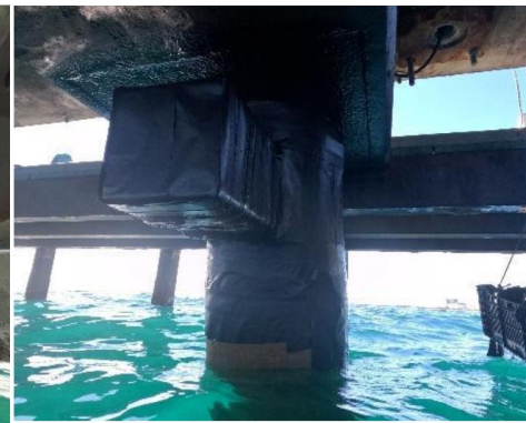
Pile Cap Paint and Pile Wrapping
