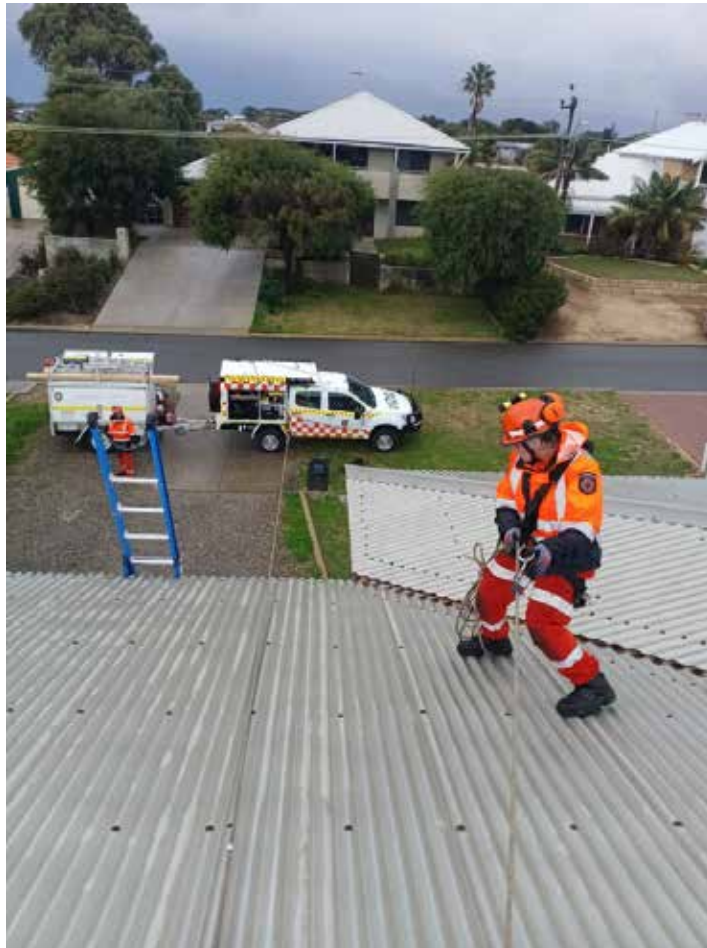
Photo: SES assessing roof damage - weather event 24 August 2025
