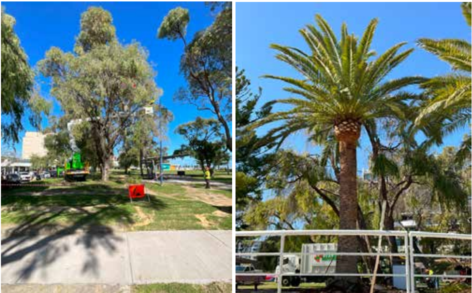
Tree Pruning Works – Churchill Park
