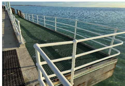
Re-installation of painted handrails
