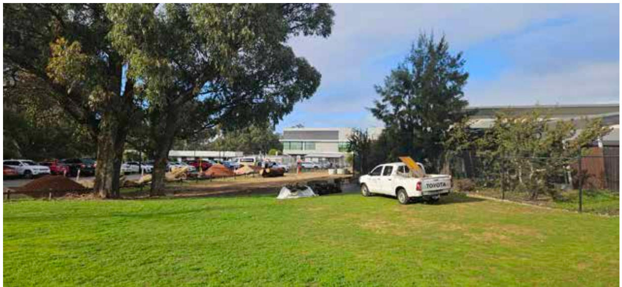
Monday 4 August 2025 - Day 1: The area was cleared ready for the landscape design
