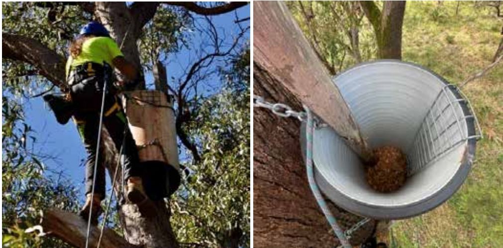
Contractor undertaking maintenance of artificial hollow
