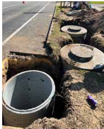
Drainage works at Safety Bay Road
