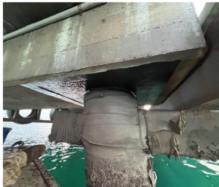
Pile Cap Paint and Pile Wrapping
