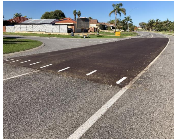
Left hand image - Image above depicts speed plateau on The Avenue and Bristol Street intersection
