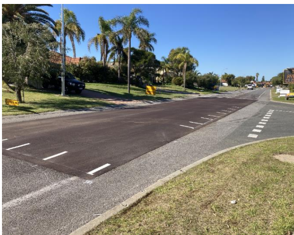
Left hand image - Image above depicts speed plateau on The Avenue and Bristol Street intersection
