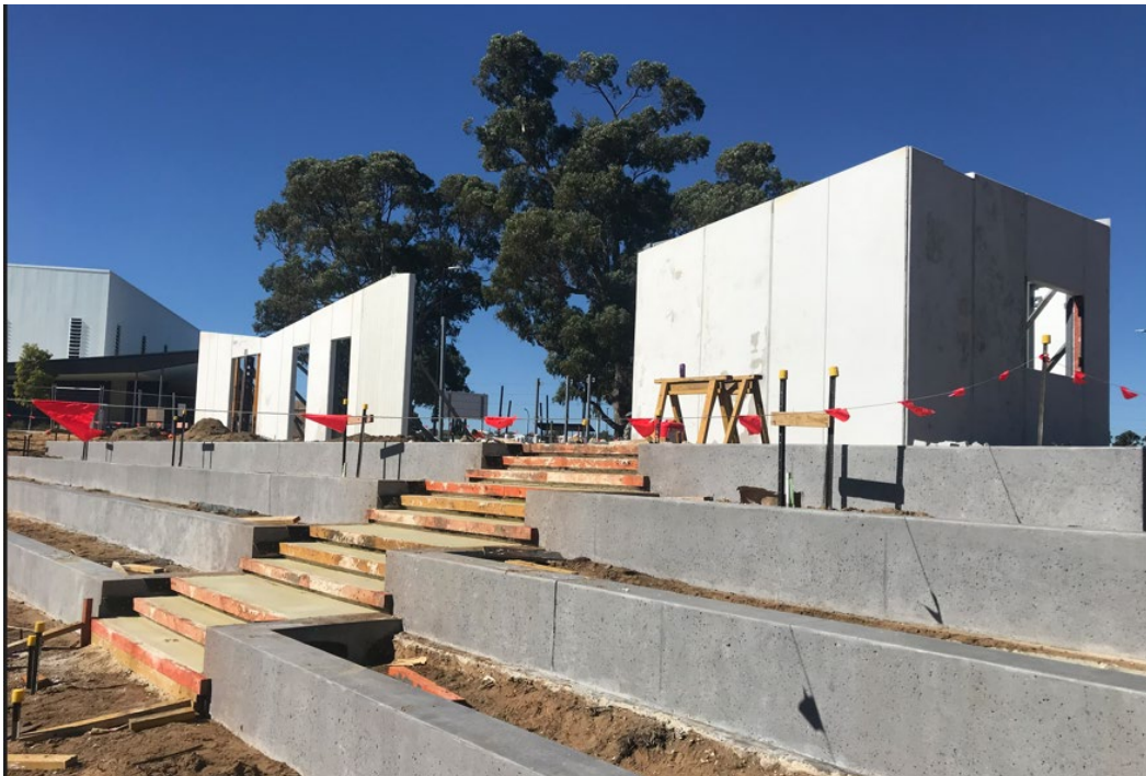
Photo 1: Baldivis Sports Complex – Southern Pavilion tilt-up panel installation
