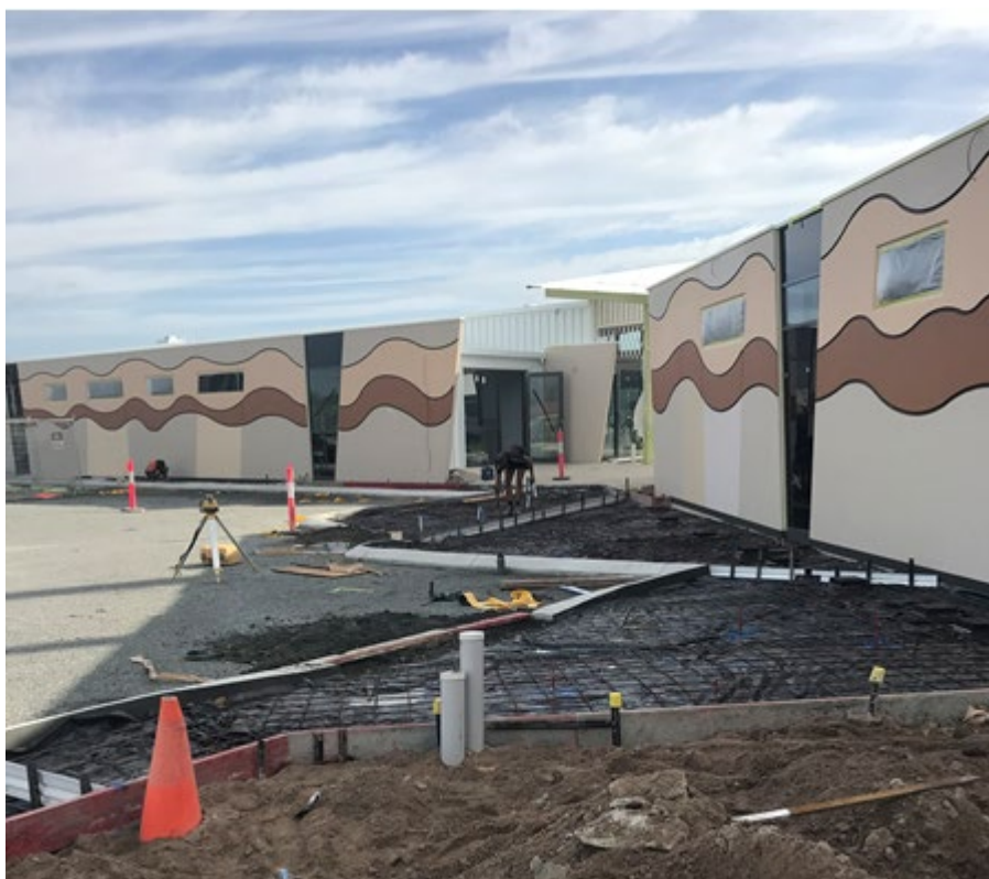
Photo 1: Stan Twight Reserve Clubroom Redevelopment – car park works kerbing and pedestrian pathway set out
