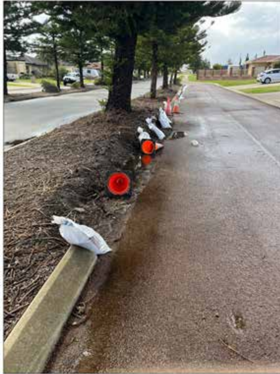
Figure 1: Damaged kerb has been removed outside 55 Chelmsford Ave Port Kennedy.
