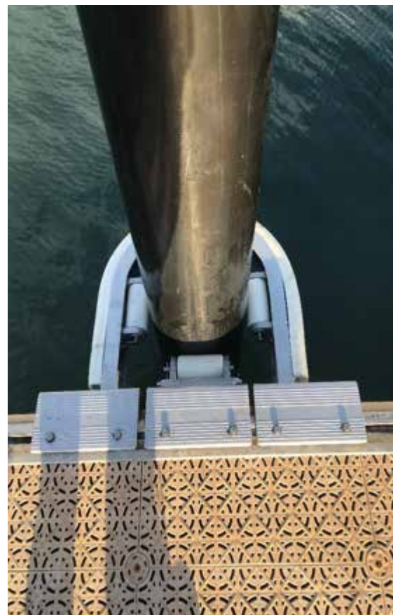
Point Peron Stakeholder Pontoon Pile Guide Bracket Replacement – May 2024
