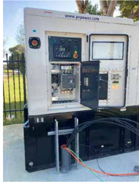
Connecting the generator
