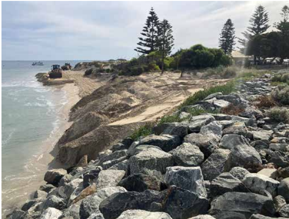
Sand placement at Mersey Point's southern beach
