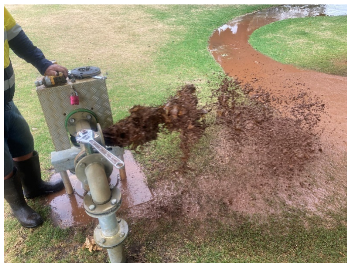
Flushing of bore iron deposits, Baldivis
