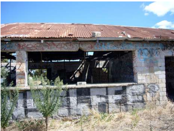
Photo 15 Partial view of eastern of east elevation of the dairy showing missing column to the opening and failure to beam
