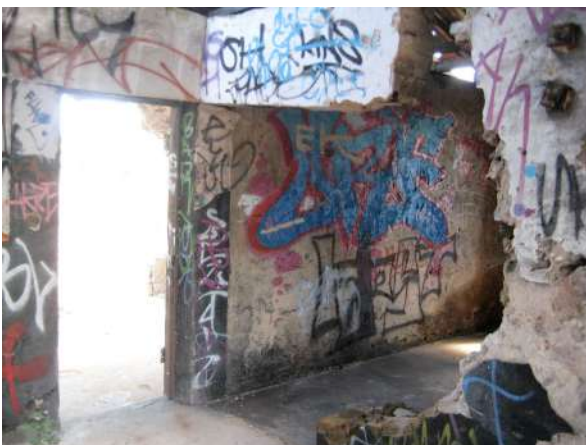
Photo 29 Internal view showing collapsed portion of wall to the door opening and failure to the beam in Room B
