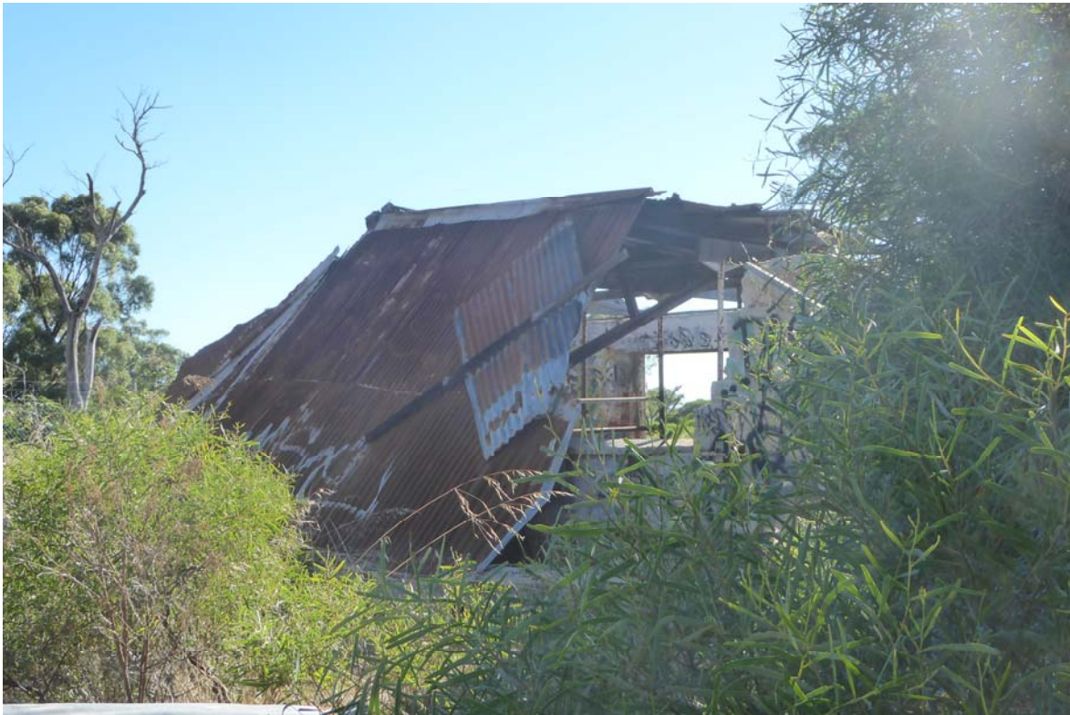
Figure 10 Collapsed roof to the East
