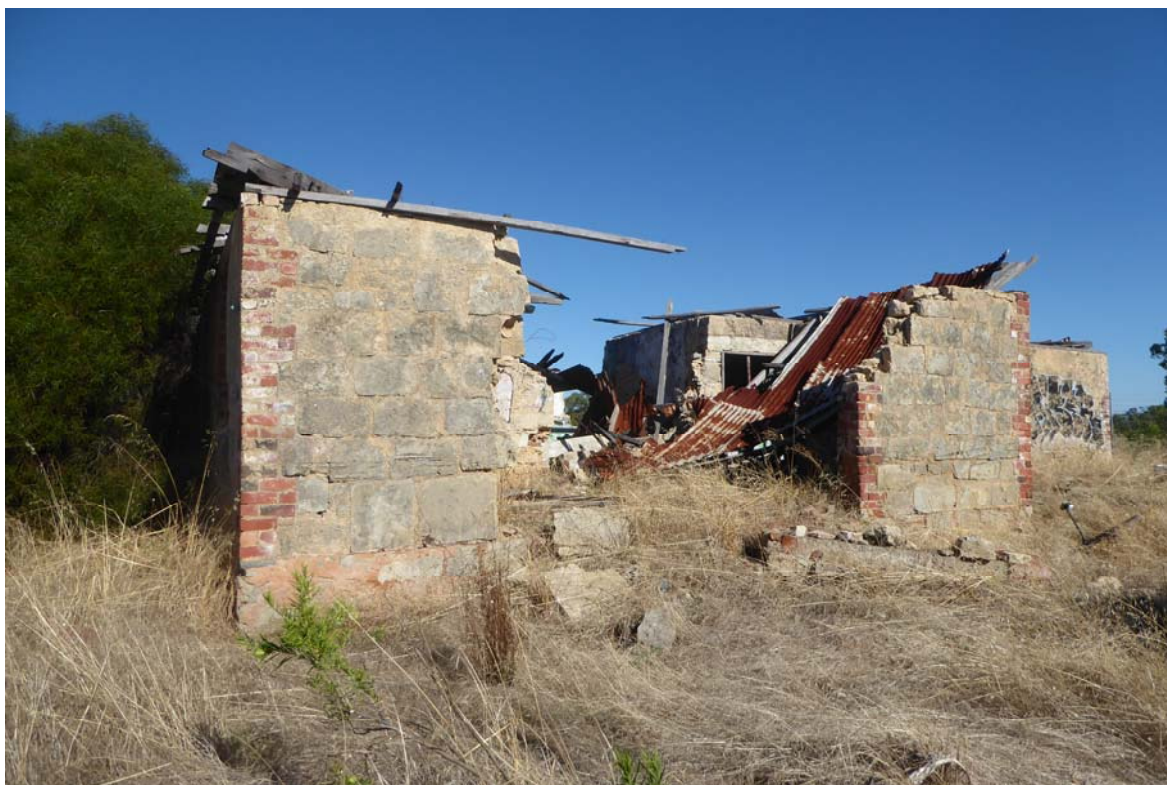
Figure 8 Partially collapsed walls and remnants of the roof
