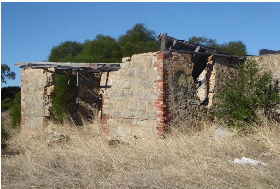
Figure 5 Partially collapsed walls of the Dairy
