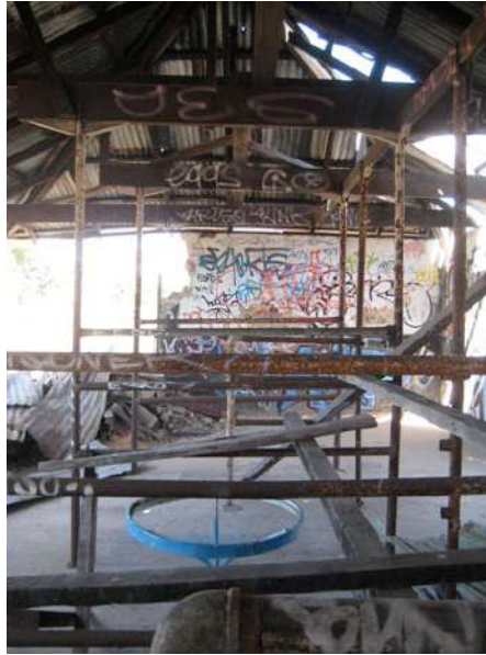
Photo 14 Detail view of tubular metal milking stalls and timber roof frame in the milking room
