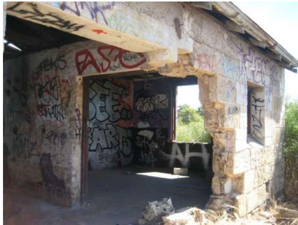
Photo 16 View showing the collapsed portion of eastern wall
