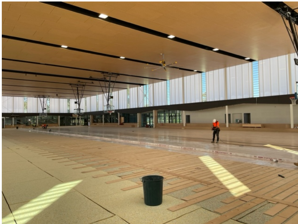
Indoor Sports Complex, installation of sports court flooring – Baldivis Sporting Complex, Baldivis
