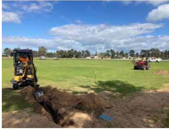
Hourglass Reserve - infield irrigation installation
