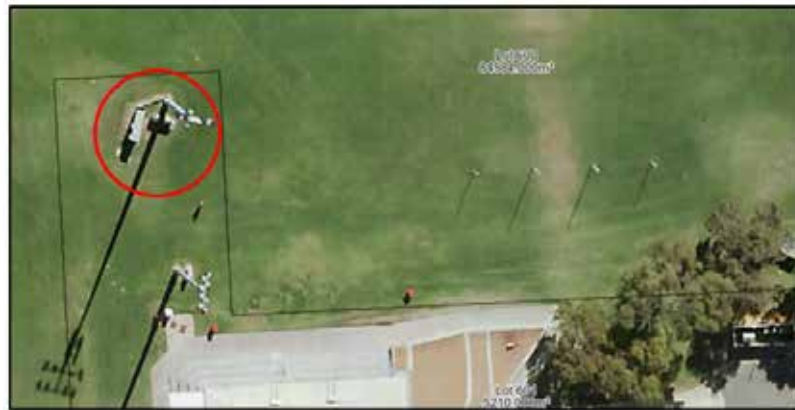
2. Leased telecommunications infrastructure and licenced flood light and associated electrical supply box shown within red circle
