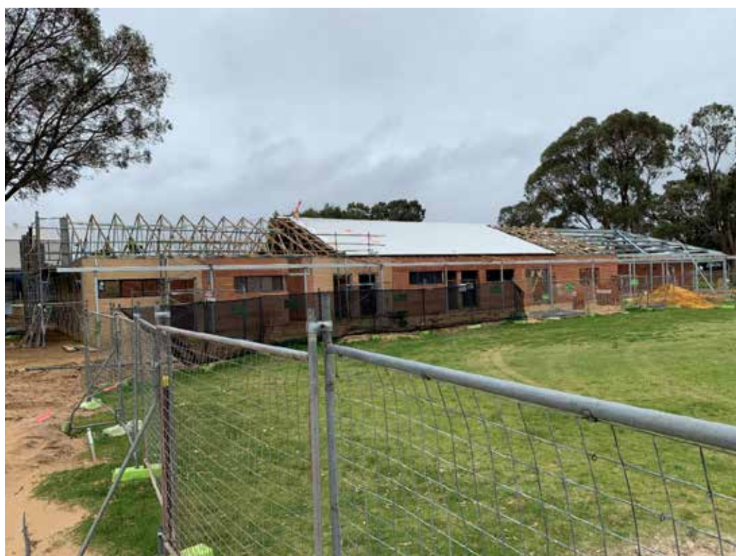
Timber roof trusses and structural steel installation – Koorana Reserve Master Plan, Warnbro
