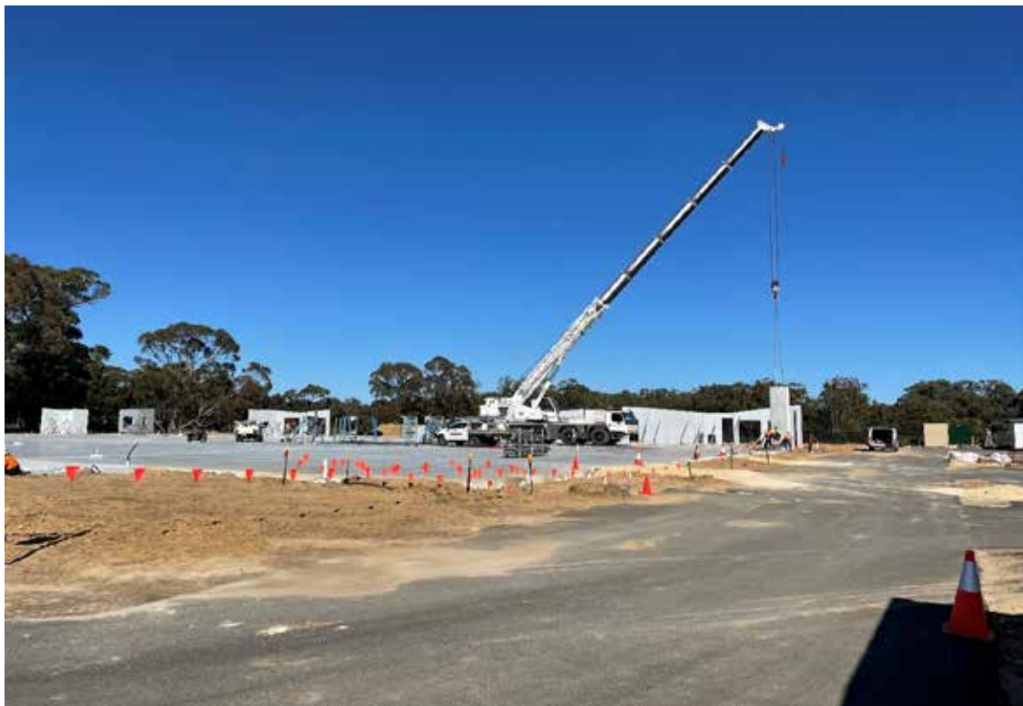
Indoor Rec Centre precast panel installation – Baldvis District Sporting Complex, Baldvis
