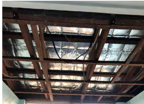
Removed asbestos sheeting from eaves and internal ceilings
