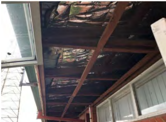
Removed asbestos sheeting from eaves and internal ceilings
