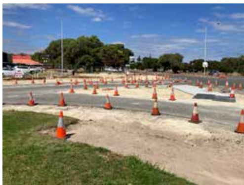
Works on Commodore Drive
