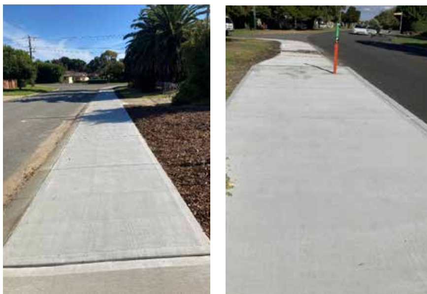
Works in progress
