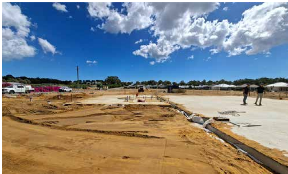
Photo 1: Baldivis Men's Shed – completion of concrete slab
