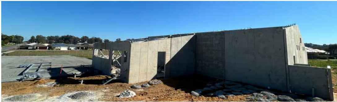
Photo 1: Baldivis Men's Shed – installed tilt up panels
