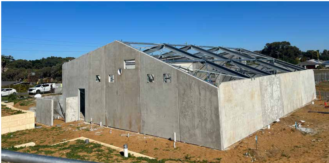
Photo 2: Baldivis Men's Shed – installed perimeter steelwork
