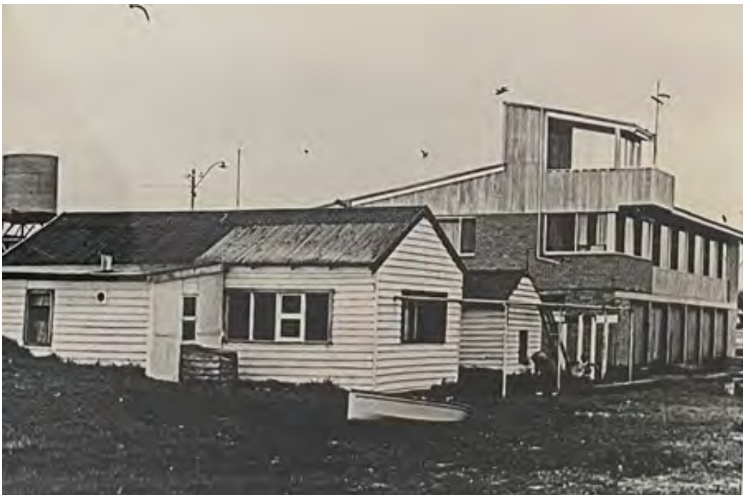
Figure 8 Safety Bay Yacht Club in the 1970s with asbestos cement roofing and wall cladding, with the 1949 buildings in the foreground. This was taken prior to the addition of the female toilets and change rooms to the west. Courtesy City of Rockingham.
