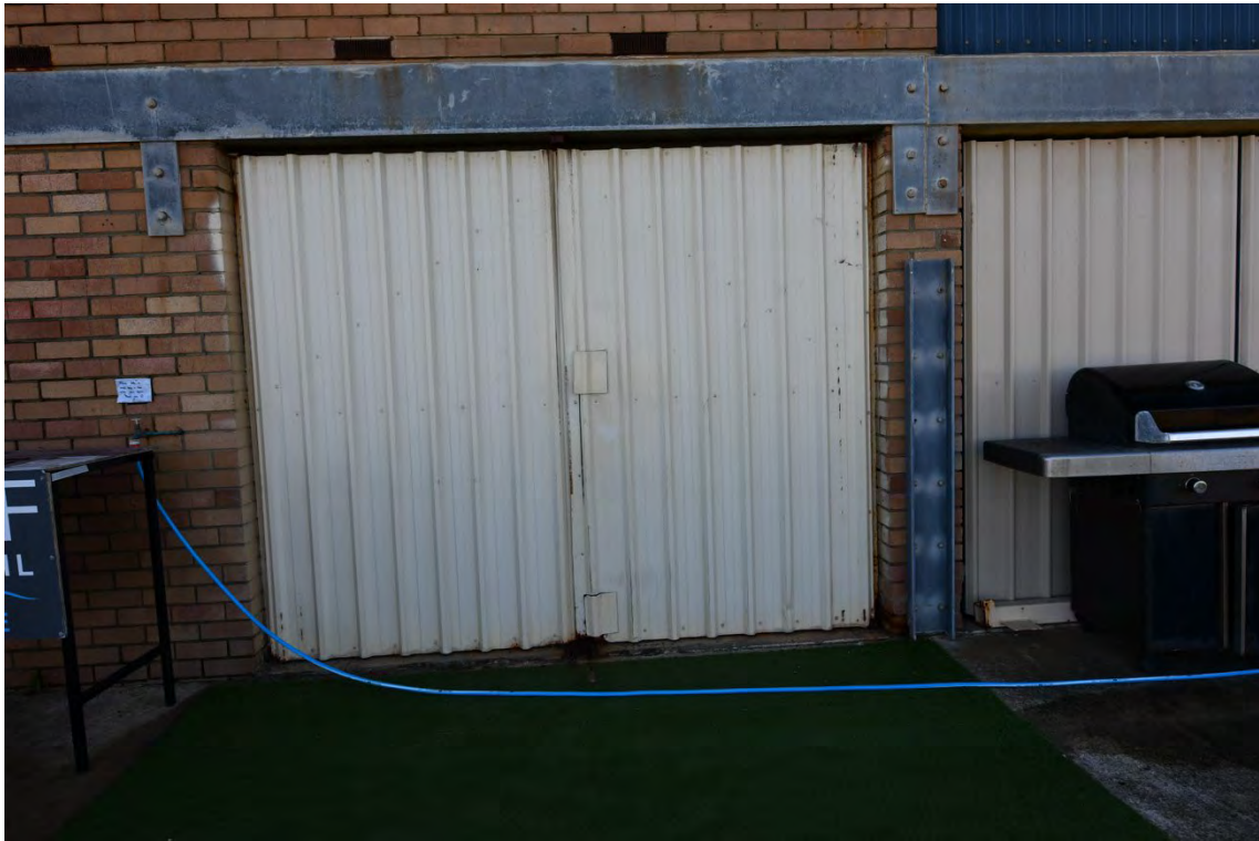
Photograph 7 Detail of pier stiffening repairs and lintel repairs. Griffiths Architects, May 2026
