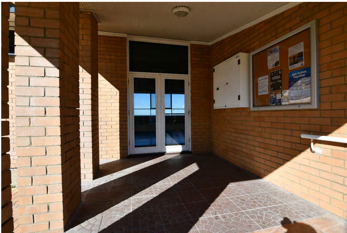
Photograph 6 Main entrance to the club rooms. Griffiths Architects, May 2026.
