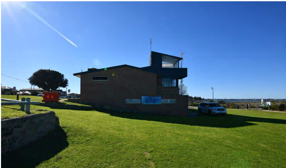
Photograph 2 View from the west showing the changeroom and toilet addition. The vertical cladding was originally asbestos cement and was replaced with corrugated steel. Griffiths Architects, May 2026.
