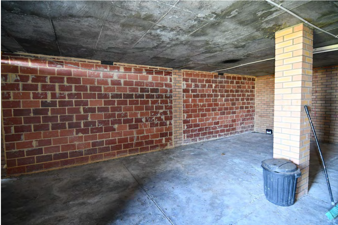
Photograph 18 West end of the boat store. Griffiths Architects, May 2026.
