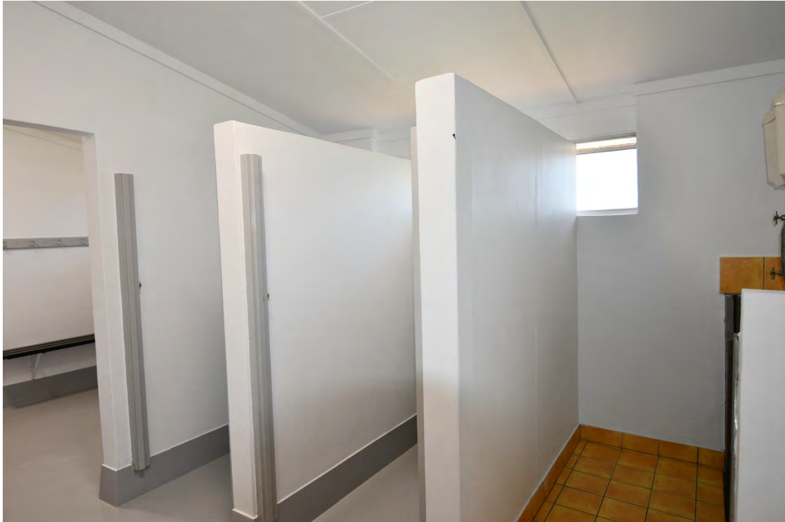
Photograph 10 Internal view of men's change rooms and showers. Griffiths Architects, May 2026.
