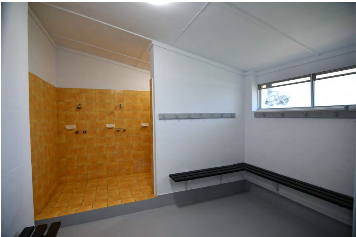
Photograph 11 Men's change rooms and showers. Griffiths Architects, May 2026.
