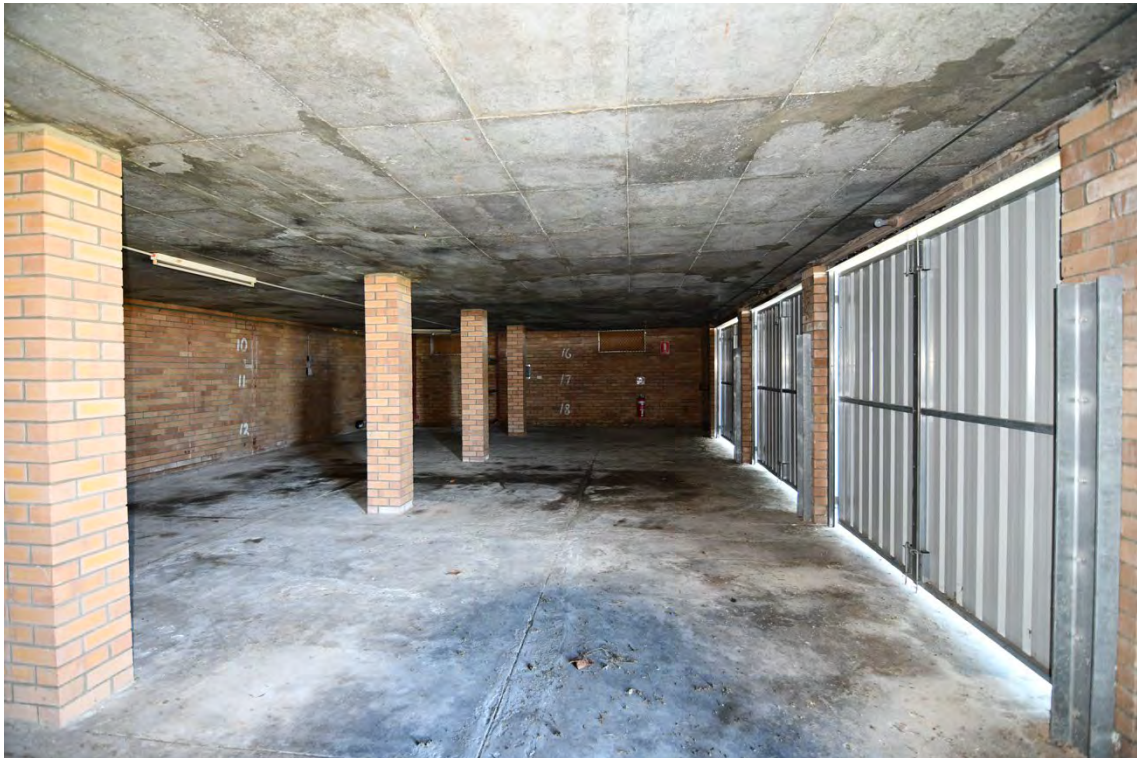
Photograph 19 Boat store looking east. Griffiths Architects, May 2026.
