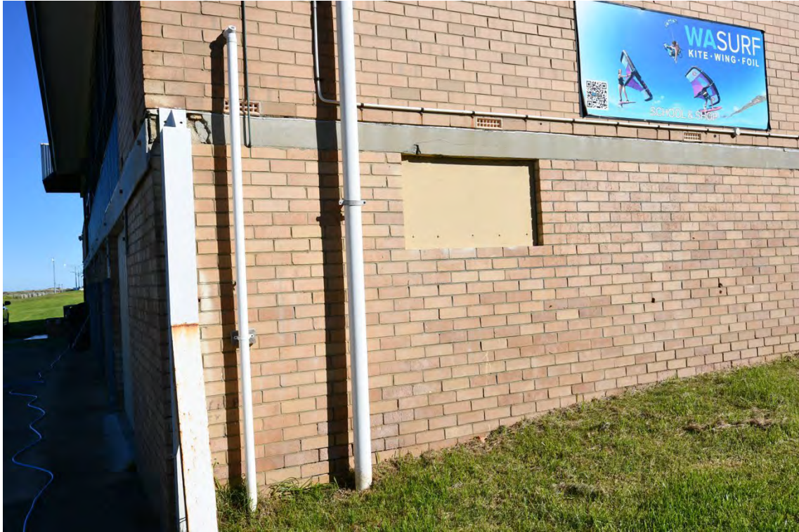
Photograph 5 Detail of structural repairs to south east corner. Griffiths Architects, May 2026.
