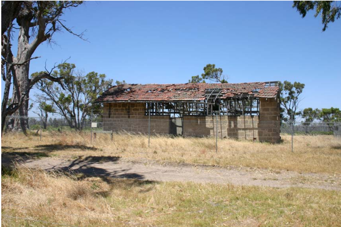
Figure 20: Old Abattoir Building, Dixon Road
