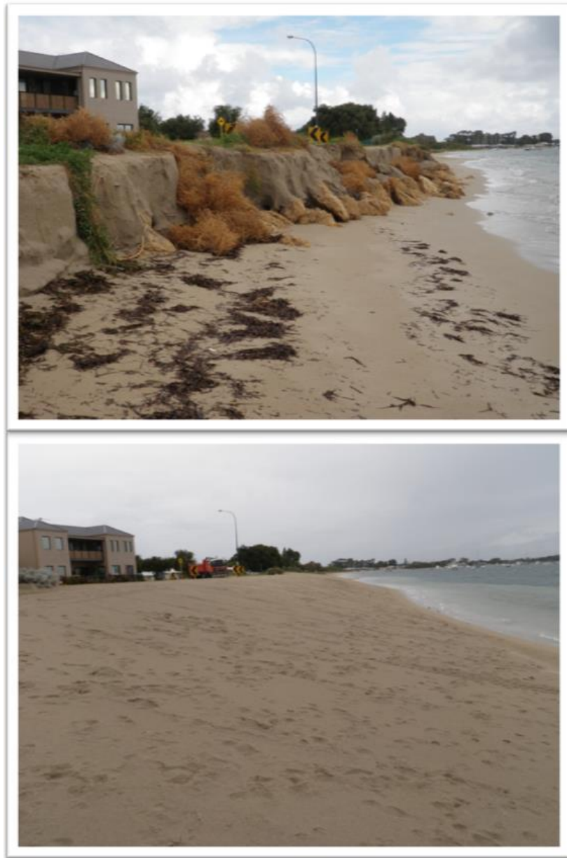
Figure 1 Hymus Street, Rockingham - erosion experienced during a winter storm [top] and the same location after earthmoving machinery was used to distribute more sand over the area to remediate the impacts of erosion [bottom]
