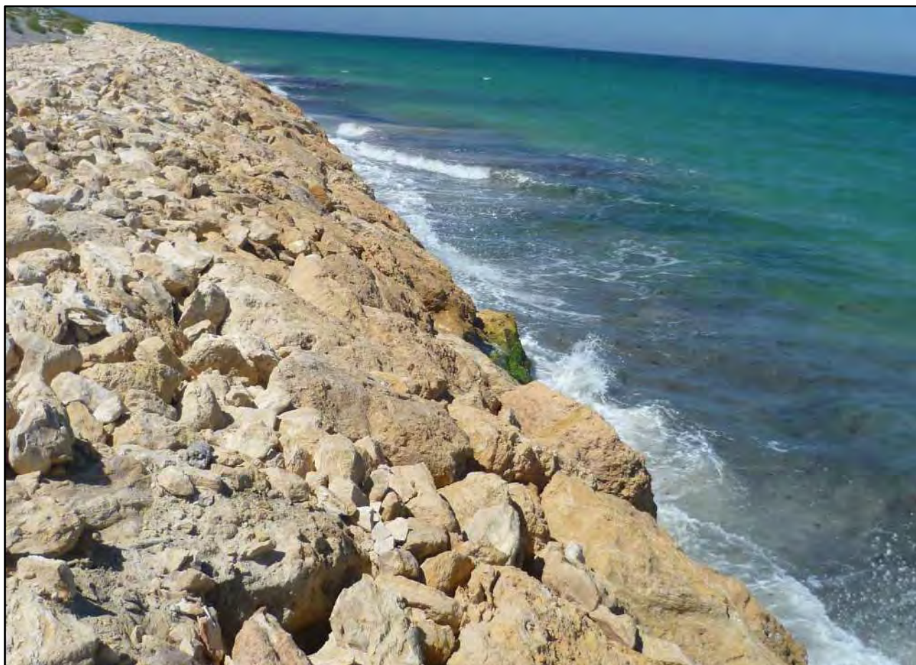
Figure 4-7 Exposed seawall where the beach in front of the seawall has been lost
