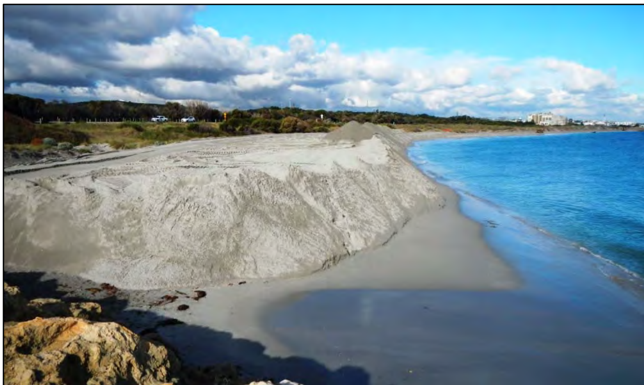
Figure 4-3 Beach renourishment occurring to advance the shoreline at C Y O'Connor Beach, North Coogee
