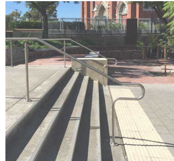
image 6.23: [HSR] Handrails to Stairs and Ramps example image, Subiaco Square
