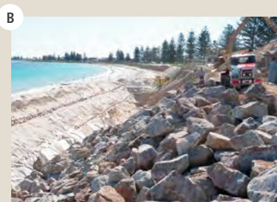
Construction of Granite Seawall
