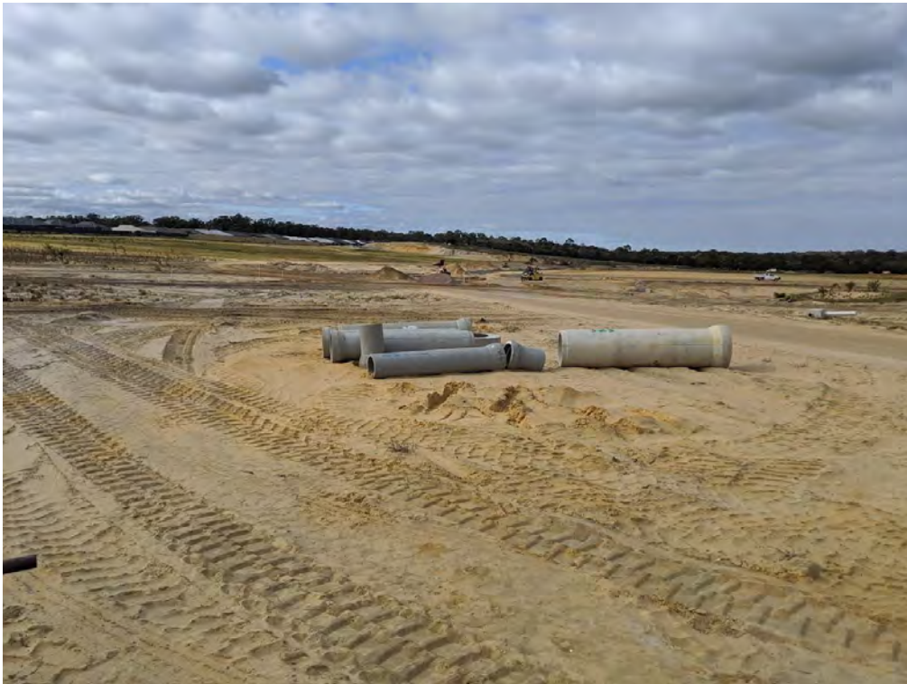
Photograph 2: General view of POS K
