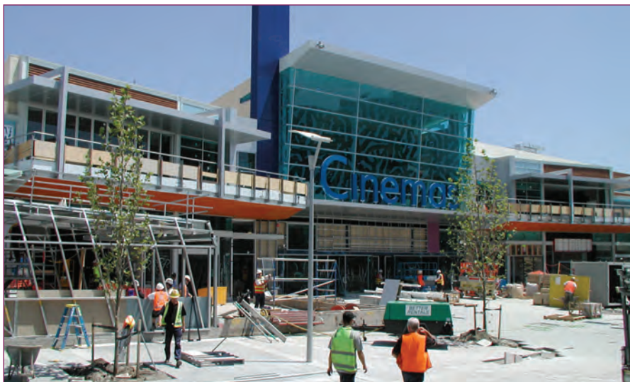
Centre elements – construction of 'main street'
