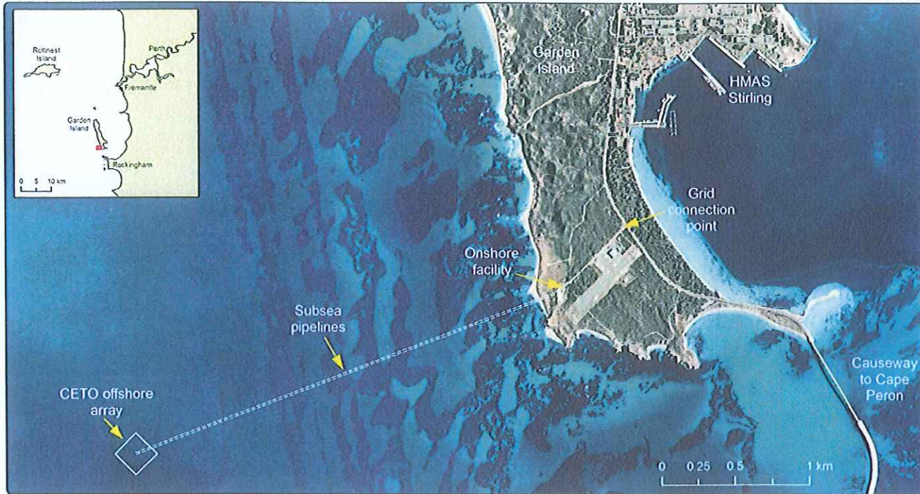
Aerial view of the Perth Wave Energy Project, Western Australia
