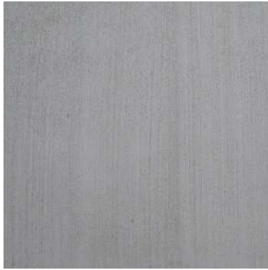
Broom finish concrete
