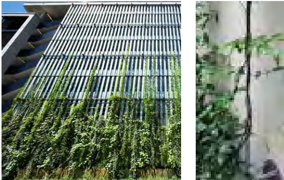
Examples of green facades with climbing plants growing on stainless steel wires.
