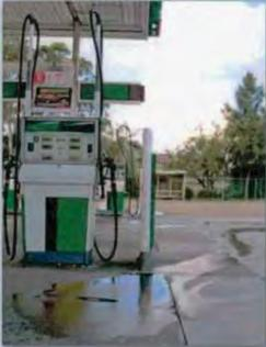
Picture shows a defective forecourt design with oils and fuels discharging directly to the street drain.
