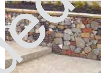
SEATING WALL Gabion Wall with Recycled Infill
