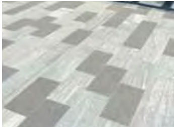
FEATURE GRANITE PAVING Granite Paving to Pedestrian Areas Size: 600x300x40mm Finish: Exfoliated
