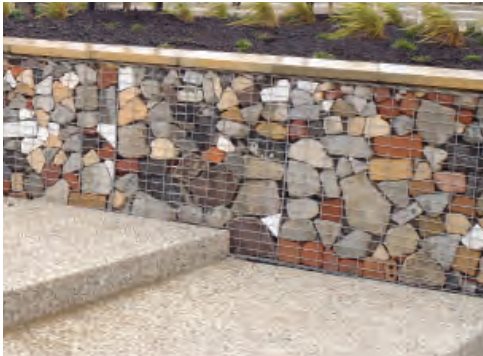
SEATING WALL Gabion Wall with Recycled Infill
