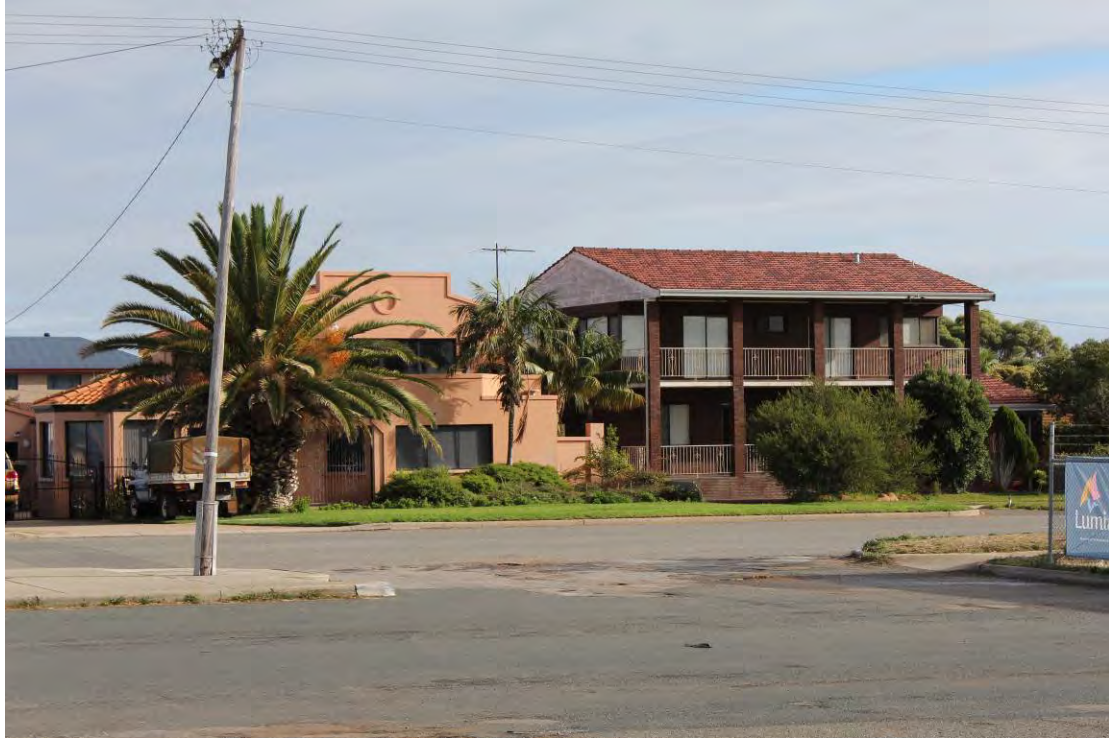
Figure 9 - View west of existing Deli on Malibu Road (R20)
