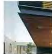
STEEL EDGE TIMBER CLADDING ON BALCONY SKIRT
