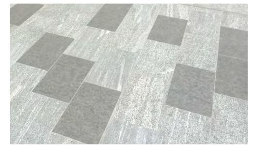
FEATURE GRANITE PAVING Granite Paving to Pedestrian Areas Size: 600x300x40mm Finish: Exfoliated
