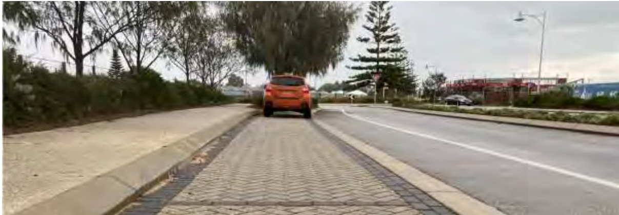
Photograph 11 – Existing parking embayment crossfall back to road on Aurea Blvd
