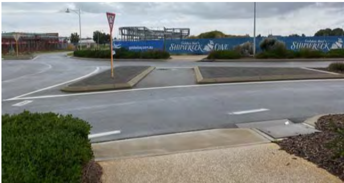
Photograph 8 – Lack of TGSIs at Aurea Blvd/ Thundelarra Dr roundabout
