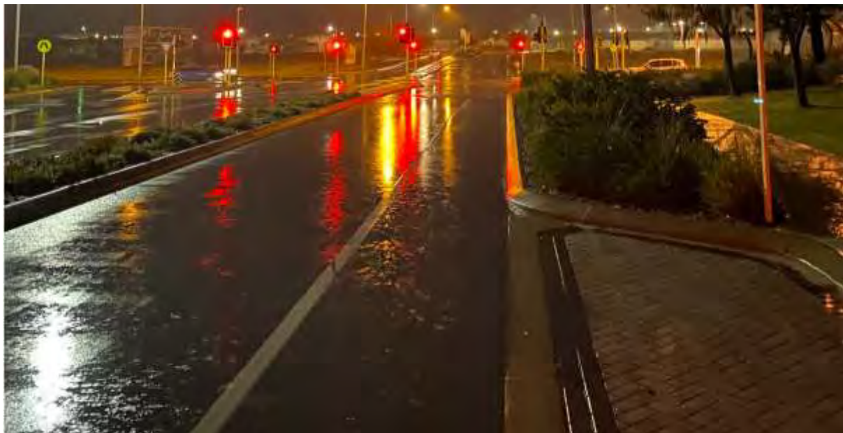
Photograph 12 – Existing parking embayment crossfall back to road on Aurea Blvd during wet conditions
