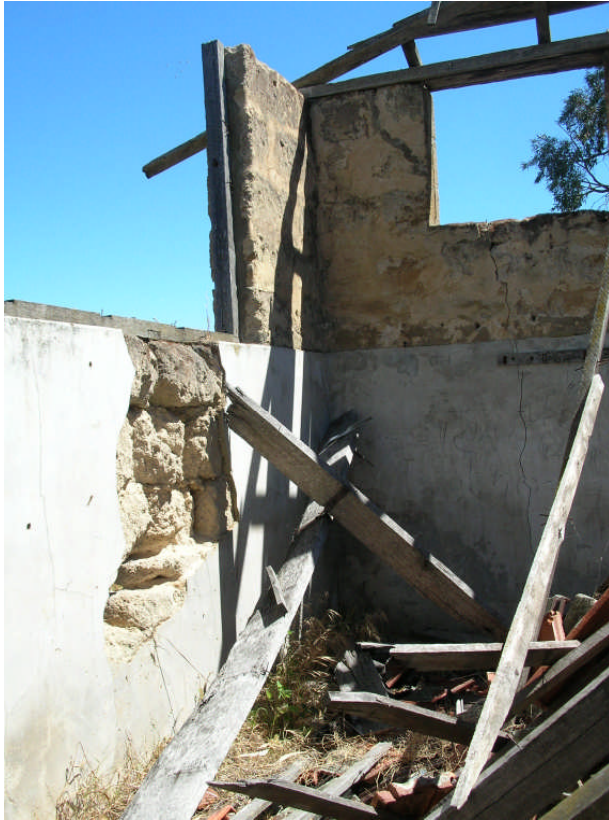
Figure 10. Damage to masonry and rendered internal face on the south-east wall. Hocking Planning & Architecture, December 2008
