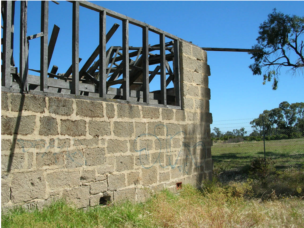
Figure 8. View of north-west wall. Floor level vents are only located within this southern section. Hocking Planning & Architecture, December 2008
