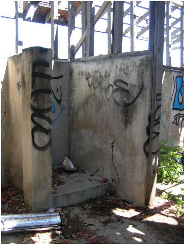
Figure 14. View of nib wall and raised concrete floor within the north room. Hocking Planning & Architecture, December 2008
