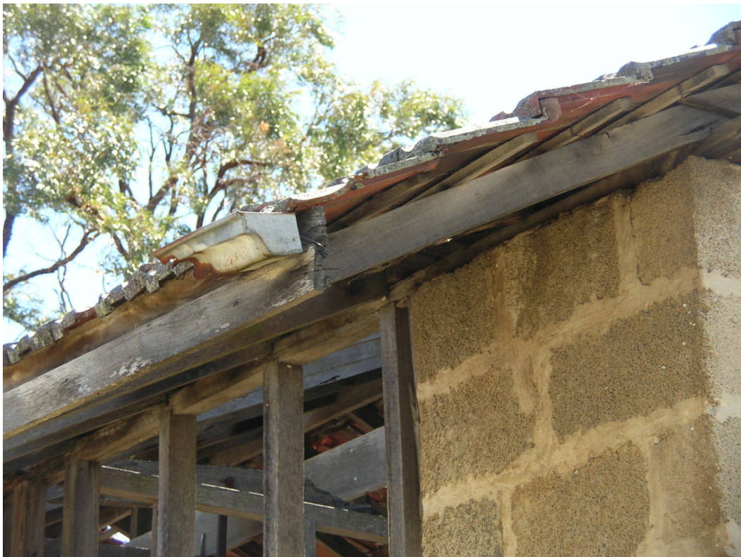
Figure 17. Remnant ogee gutter, north corner. Hocking Planning & Architecture, December 2008
