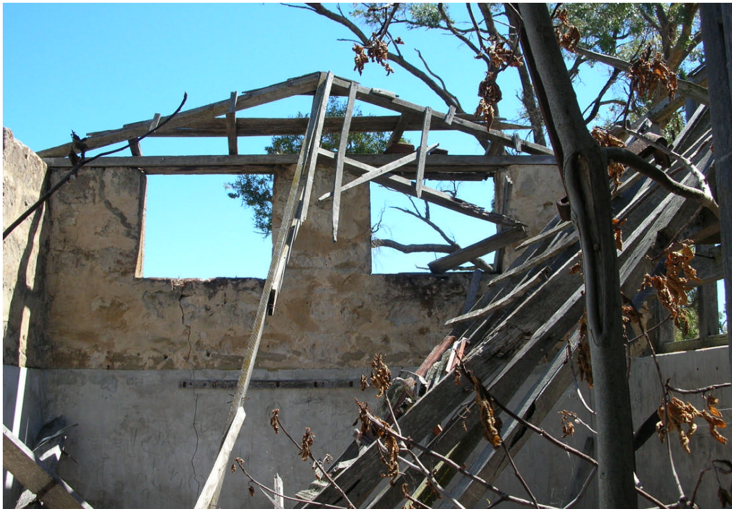
Figure 9. Internal view of the south-west wall. All that remain in this section are the limestone masonry walls. The roof structure has collapsed and remnant wall framing have deteriorated away and are at risk of collapse. Hocking Planning & Architecture, December 2008
