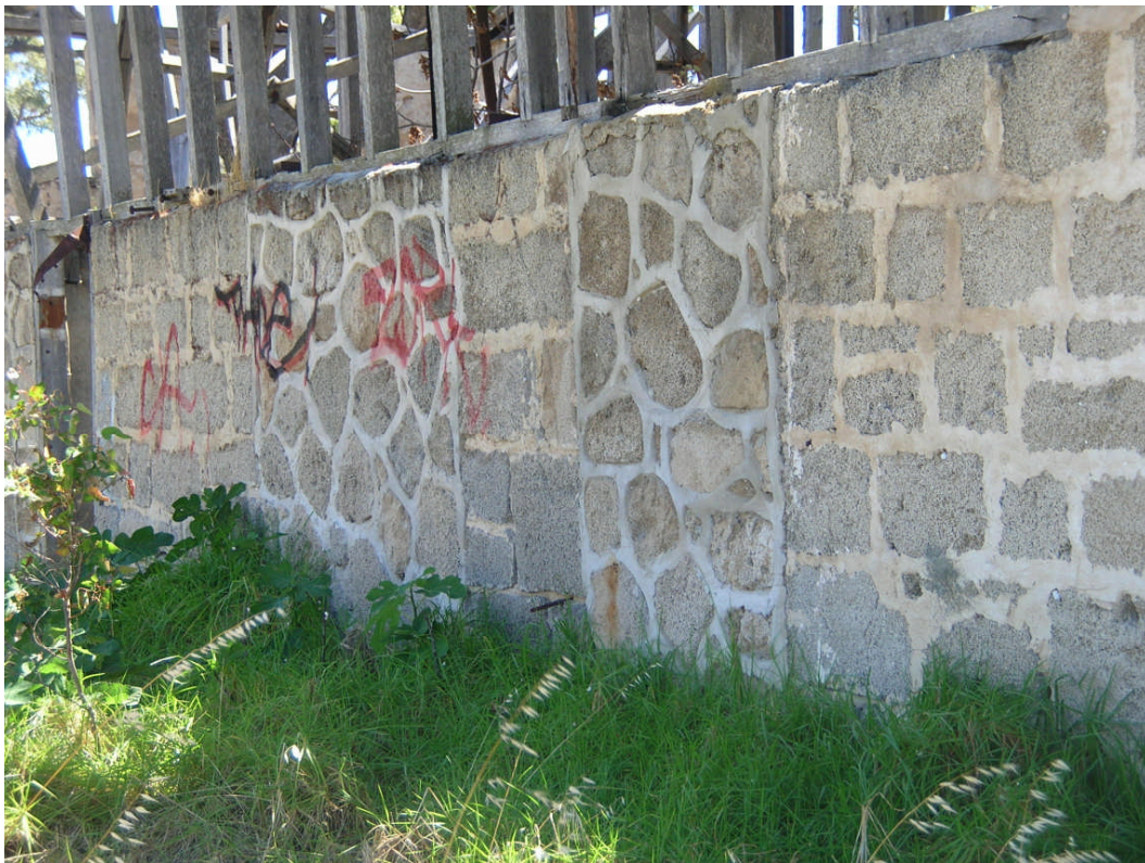
Figure 7. View of south-east wall. Note infilled sections of the wall as rubble limestone are arranged in an irregular bond. Careful removal of graffiti is required to prevent damage to the vuggy limestone surfaces. Hocking Planning & Architecture, December 2008
