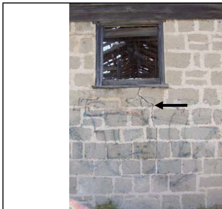
Photograph 17 – North east wall external Arrow - Cracking
