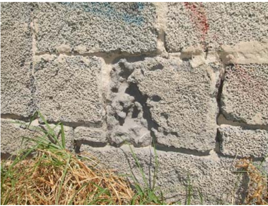
Photograph 15 – Wall erosion – north west elevation
