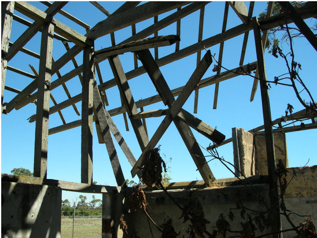
Figure 11. Internal view of the south-east wall and partially collapsed roof structure. For safety reasons, all roof and wall structure should be removed and salvaged for later reinstatement where possible. Hocking Planning & Architecture, December 2008
