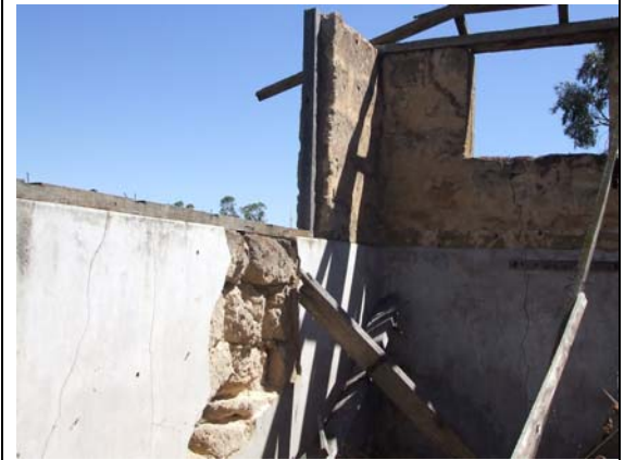
Photograph 14 – Wall erosion. Inside location of photograph 13
