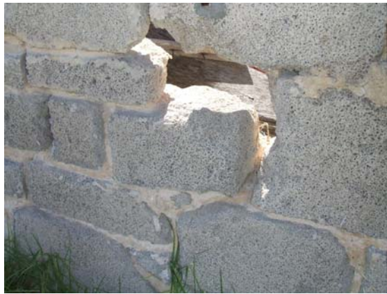
Photograph 13 – Wall erosion – South east wall
