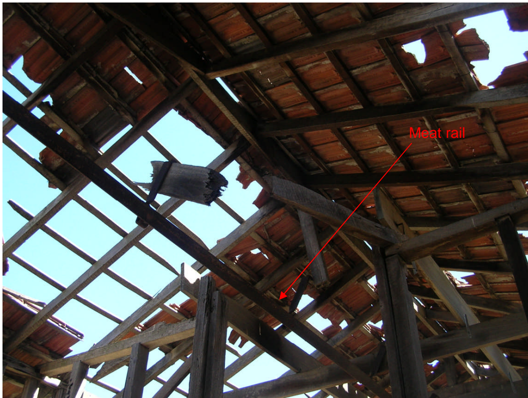
Figure 12. Underside of remnant roof structure and steel beam identified as 'meat rail' which is suspended from deteriorated timber structure. Hocking Planning & Architecture, December 2008
