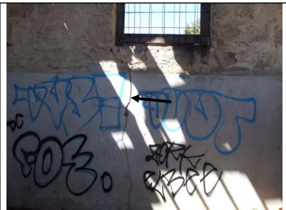
Photograph 18 – North east wall internal Arrow – cracking. Location of photograph 17
