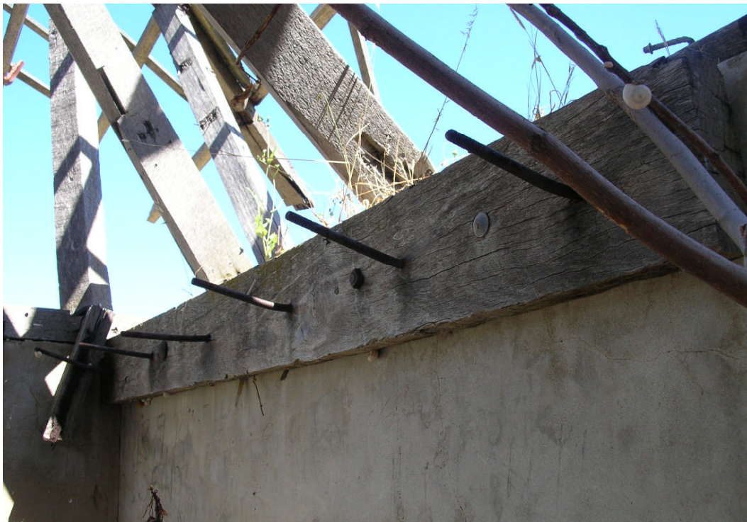
Figure 15. Detail of wall mounted timber with evenly spaced steel dowels associated with the former uses of the place. Hocking Planning & Architecture, December 2008
