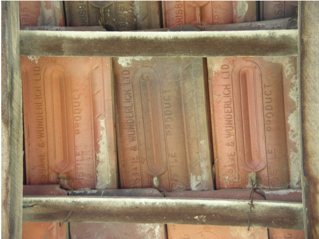
Figure 16. Detail of Marseille pattern roof tiles with maker's mark. Hocking Planning & Architecture, December 2008
