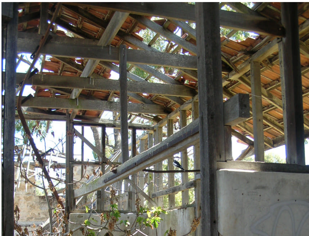
Figure 13. View of meat rail spanning the length of the central room. Hocking Planning & Architecture, December 2008
