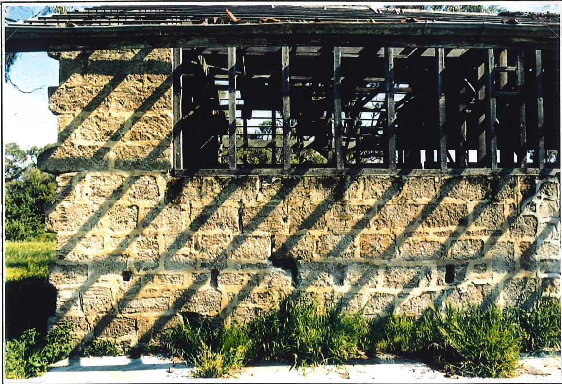
Figure 3.10 Close-up of the south-east elevation, showing the projecting key stones at the south-west end of the building, and also a line of indentations in the wall at approximately 0.55 metres above the floor level that is possibly evidence of a structure that formerly abutted this wall.
