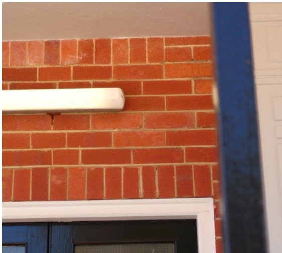
Figure 42: Vertical stretcher bricks above door entry and below ceiling
