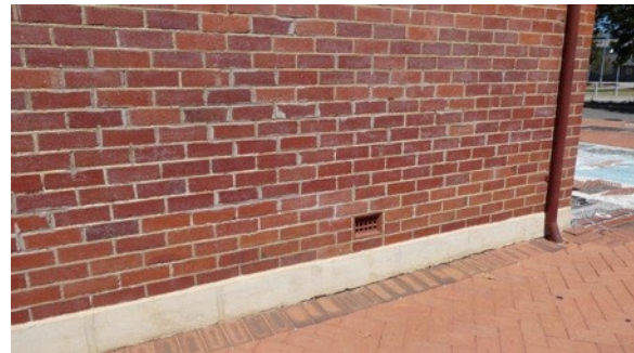
Figure 53: Stretcher bond brick construction and limestone plinth of original section
