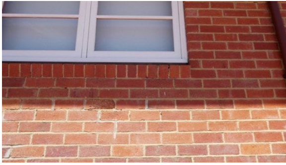
Figure 54: Angled brick sills
