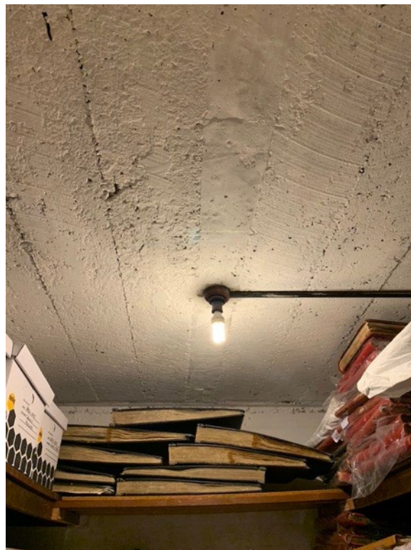
Figure 109: Reinforced concrete ceiling to Strong Room
