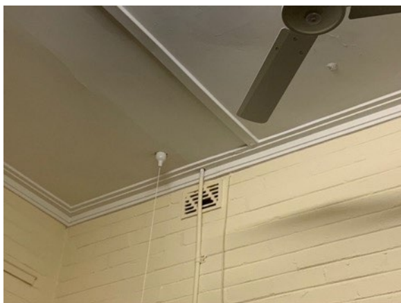
Figure 122: Painted brick walls, surface mounted conduits and pull cord light switch
