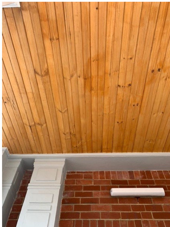
Figure 39: Pine board ceiling lining
