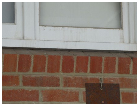
Figure 71: Angled brick window sills
