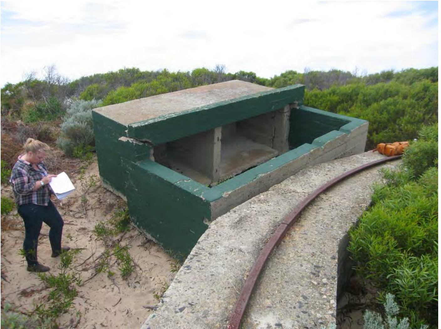
Figure 106: Gun Emplacement - Ammunition Store No. 1
