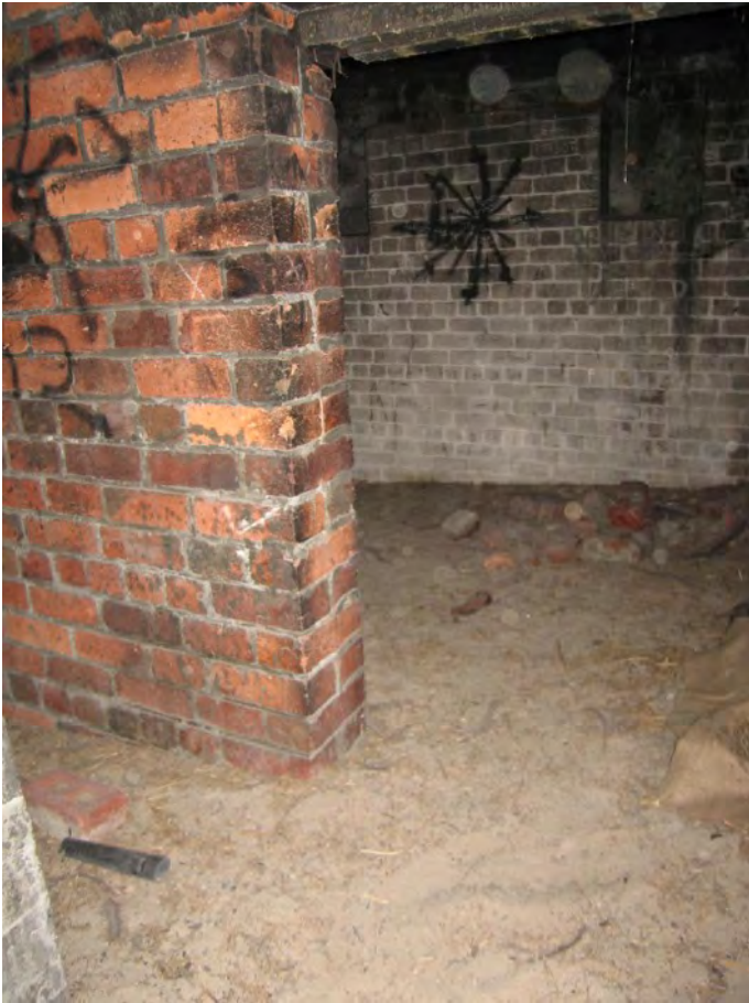
Figure 125: Ammunition Bunker – brick perimeter wall
