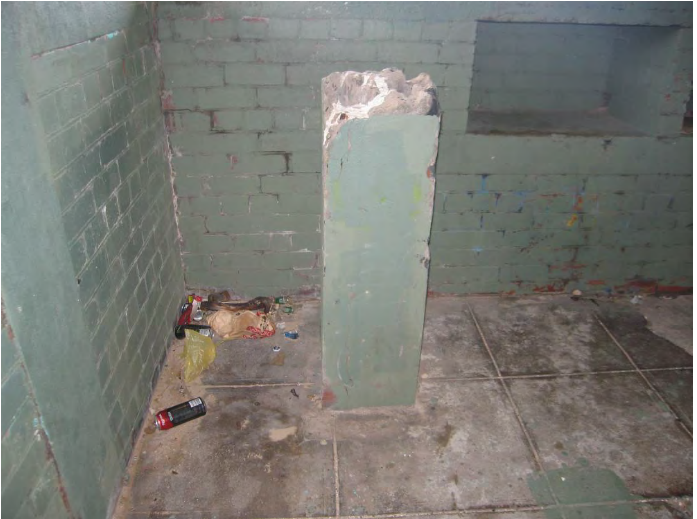
Figure 71: Reinforced concrete observation mounts
