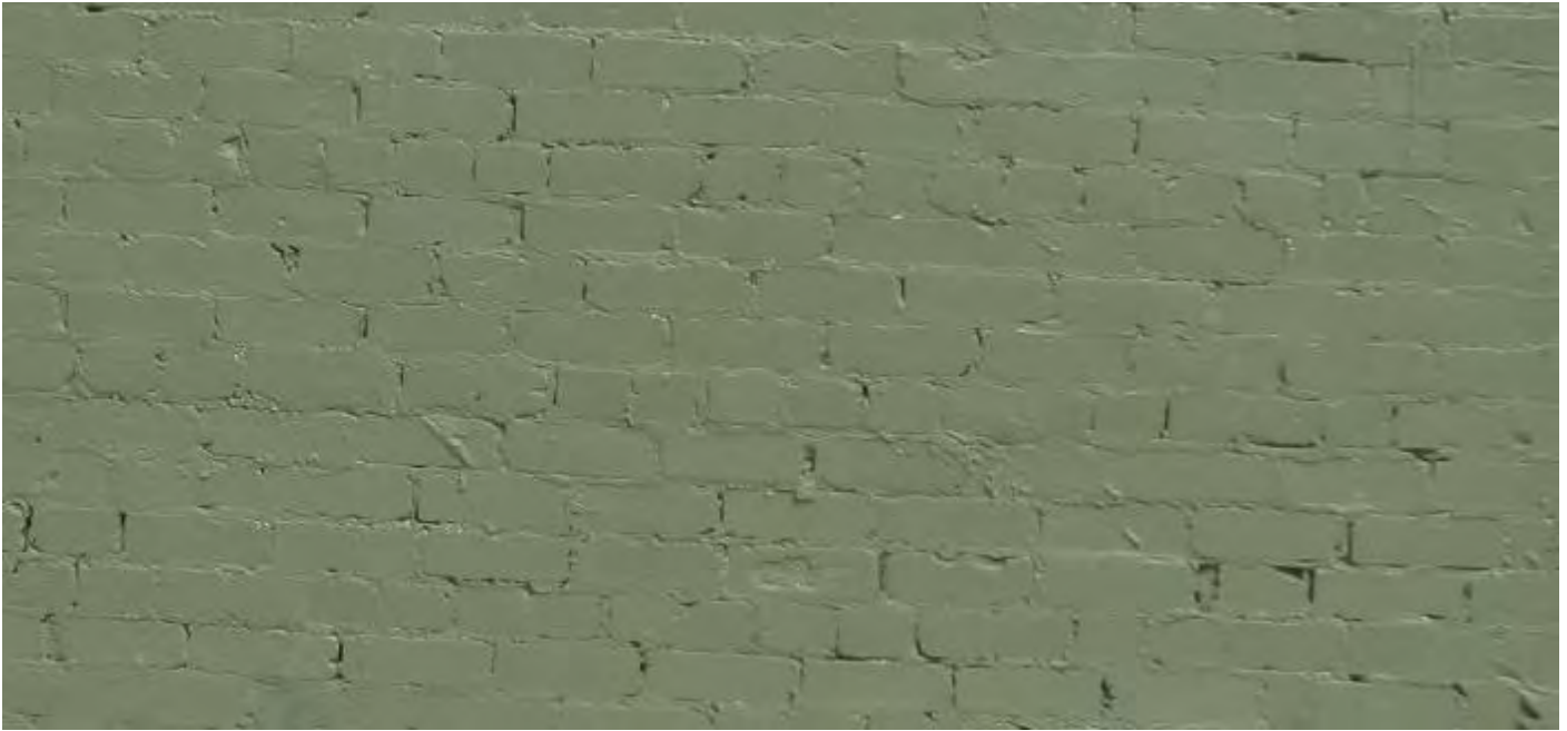
Figure 55: English Garden Bond Brickwork
