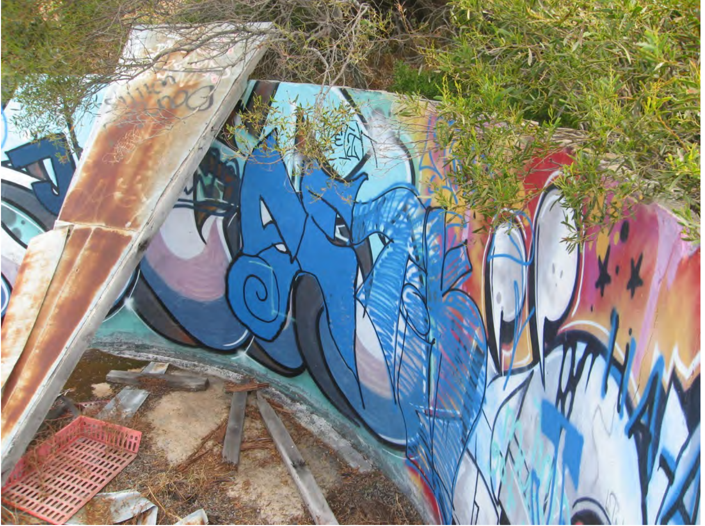
Figure 156: Water Tank Interior
