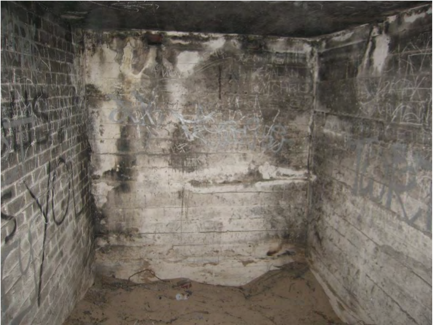
Figure 122: Ammunition Bunker – Room 1
