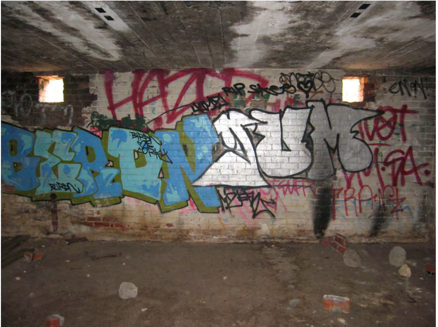
Figure 92: Operations Bunker – interior (north wall)
