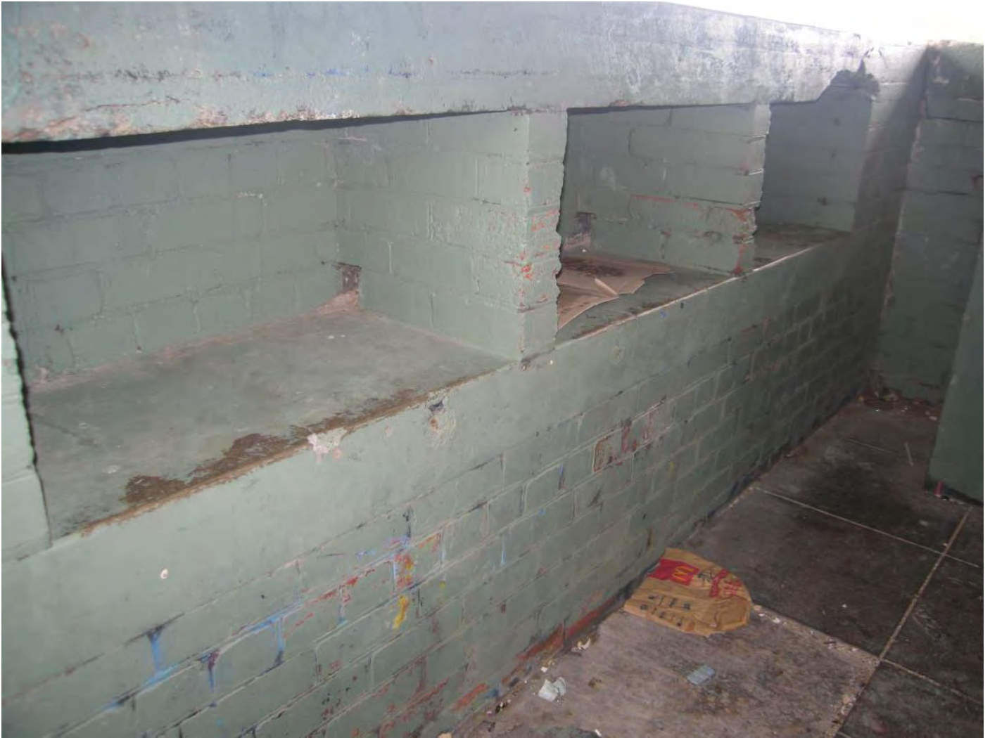
Figure 72: Storage incorporated into the west wall
