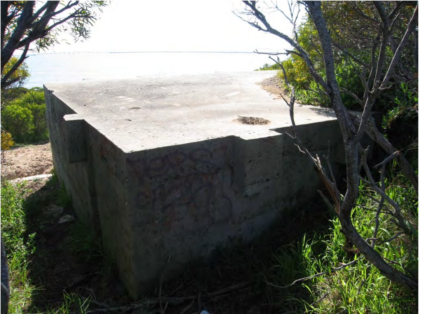
Figure 118: Ammunition Bunker – view across the roof
