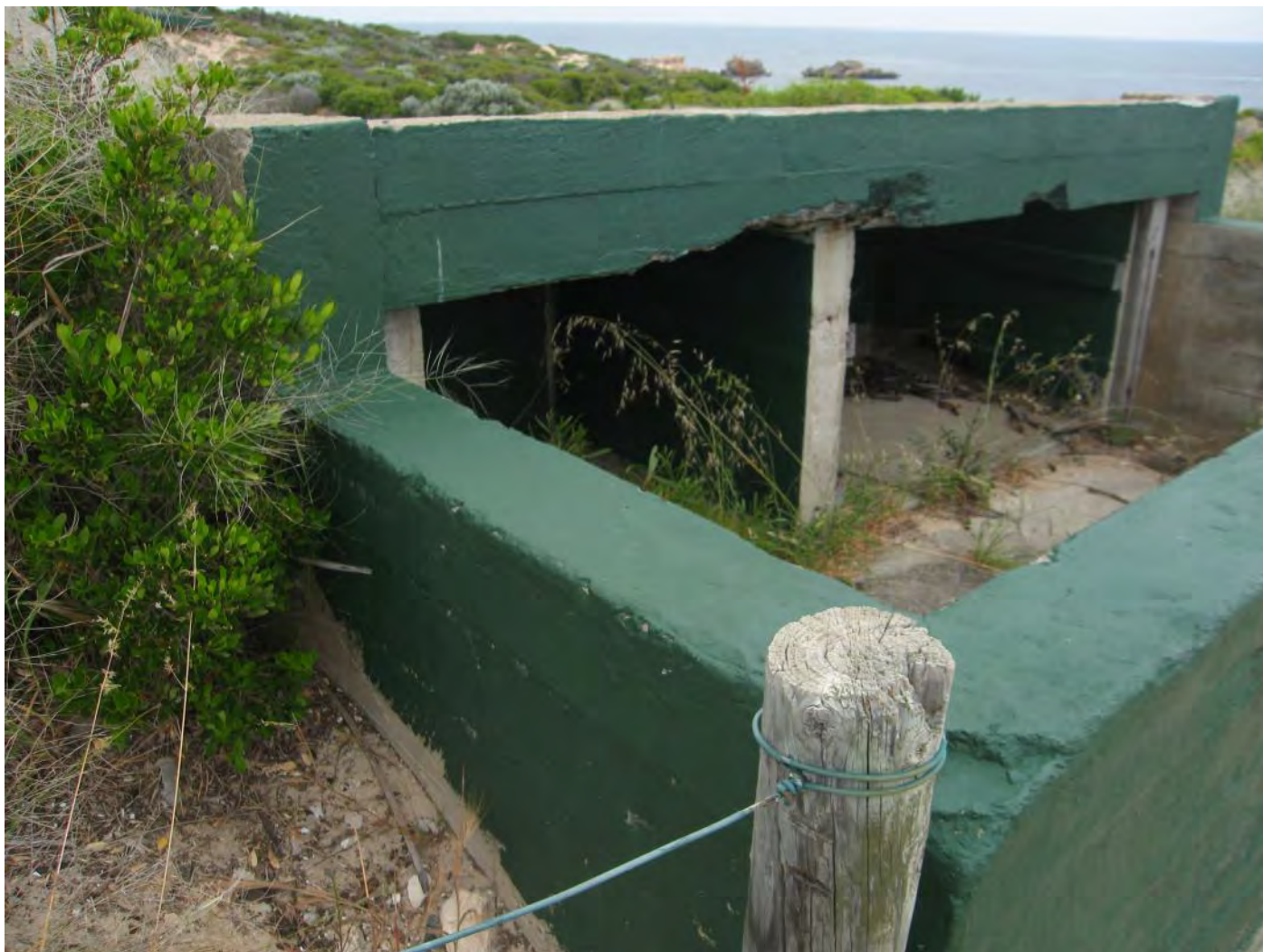
Figure 135: Gun Emplacement No. 2 – Ammunition Store 1
