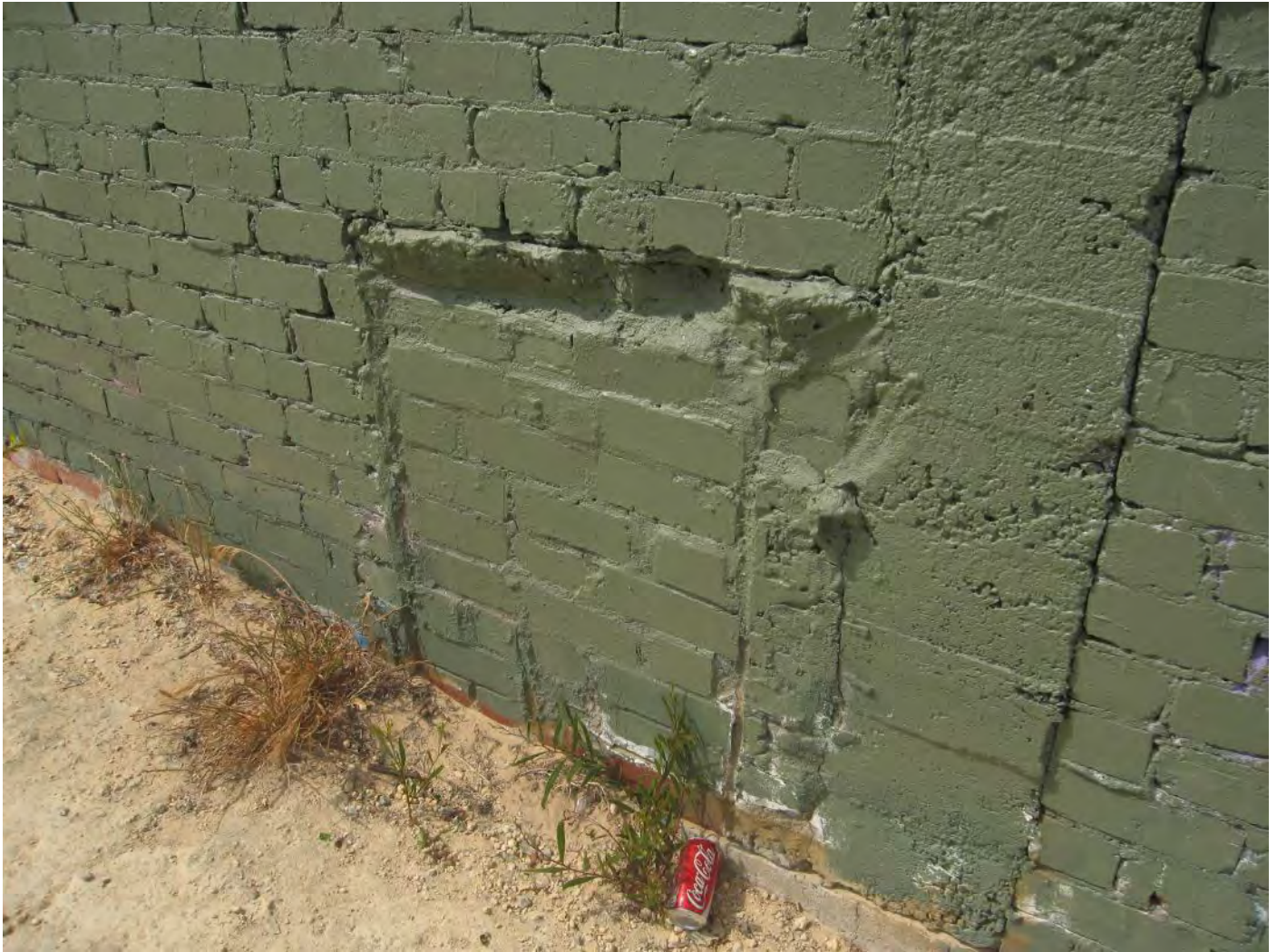
Figure 64: North Elevation – brick infill panel
