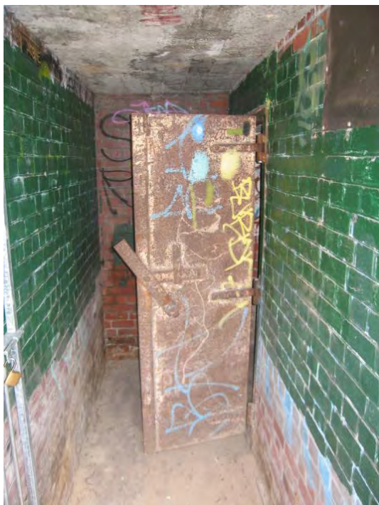
Figure 89: Operations Bunker – Extant steel entrance doors
