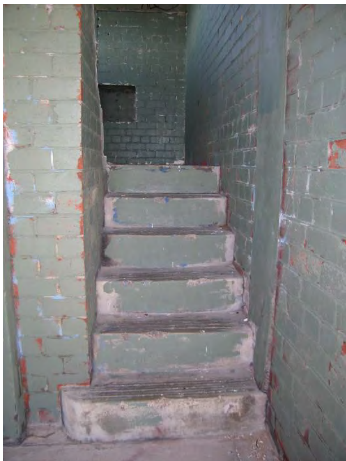
Figure 69: Stairs to upper level
