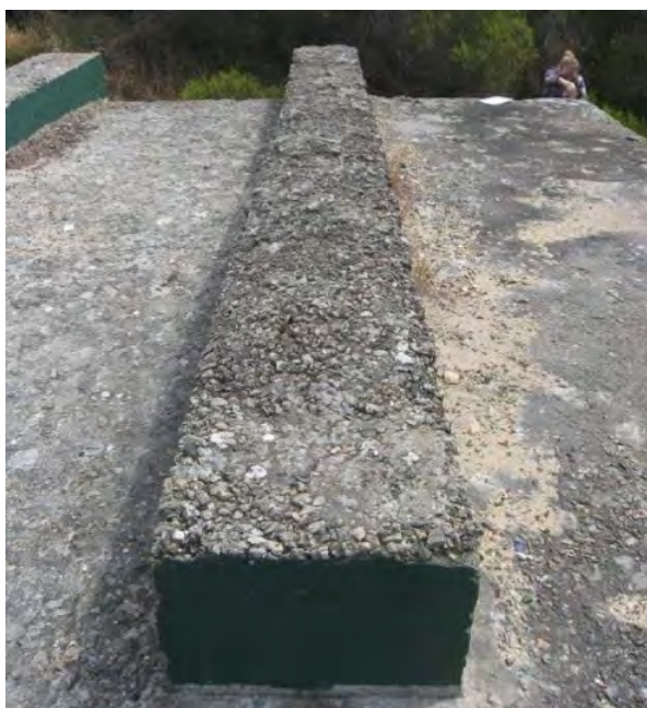
Figure 82: Operations Bunker – Reinforced concrete roof beam
