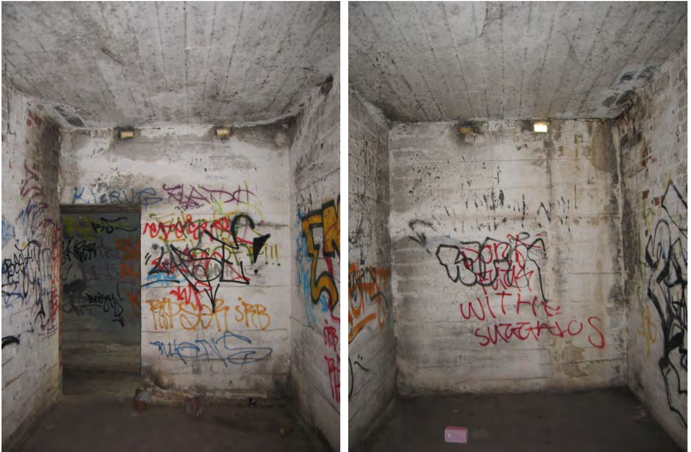
Figure 146: Ammunition Bunker - Room 1
