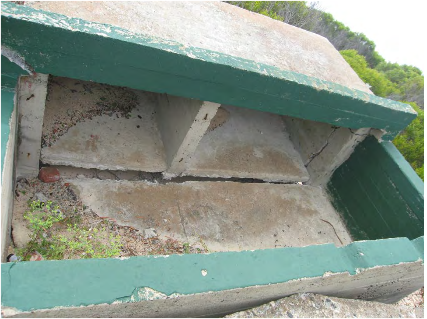
Figure 107: Gun Emplacement - Ammunition Store No. 1
