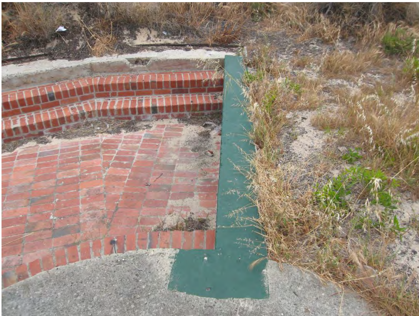
Figure 132: Gun Emplacement No. 2 – terminating concrete wall
