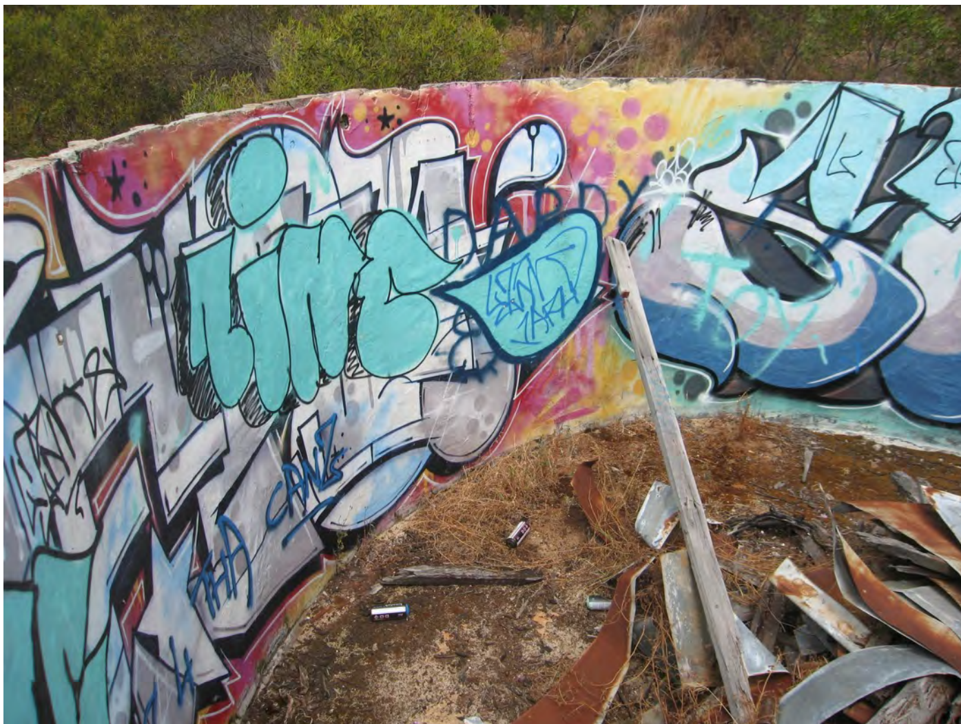
Figure 157: Water Tank interior
