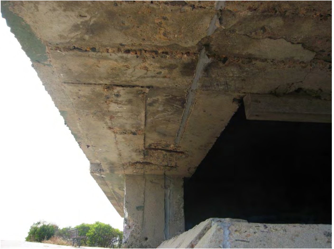
Figure 61: Underside of Concrete Overhang to Observation Opening
