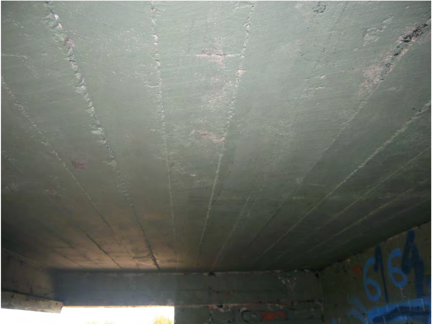
Figure 74: Concrete slab roof
