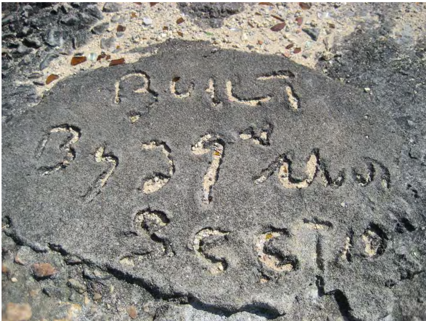
Figure 83: Operations Bunker – Roof inscription
