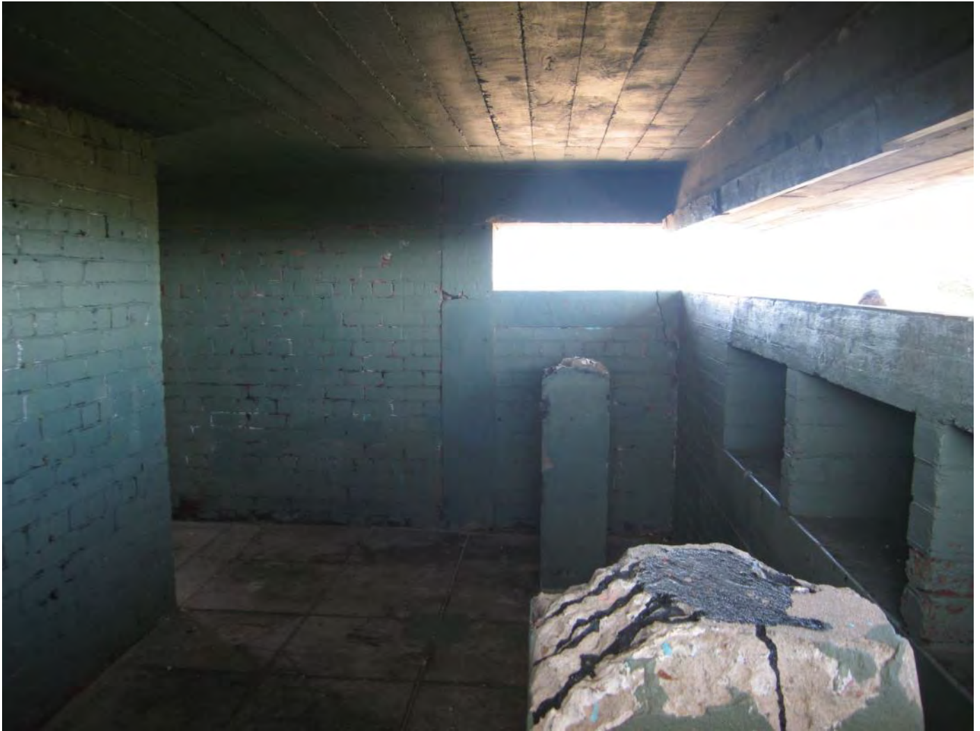
Figure 67: Ground level interior
