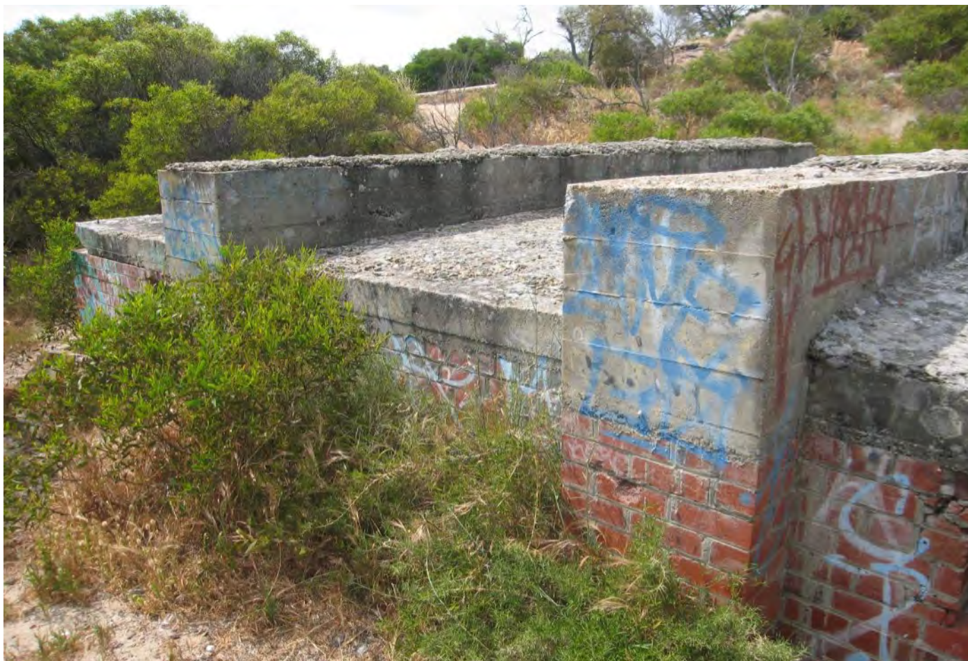
Figure 81: Operations Bunker – North wall
