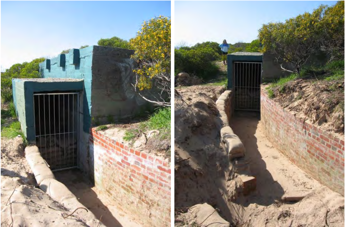
Figure 116: Ammunition Bunker - entrance
