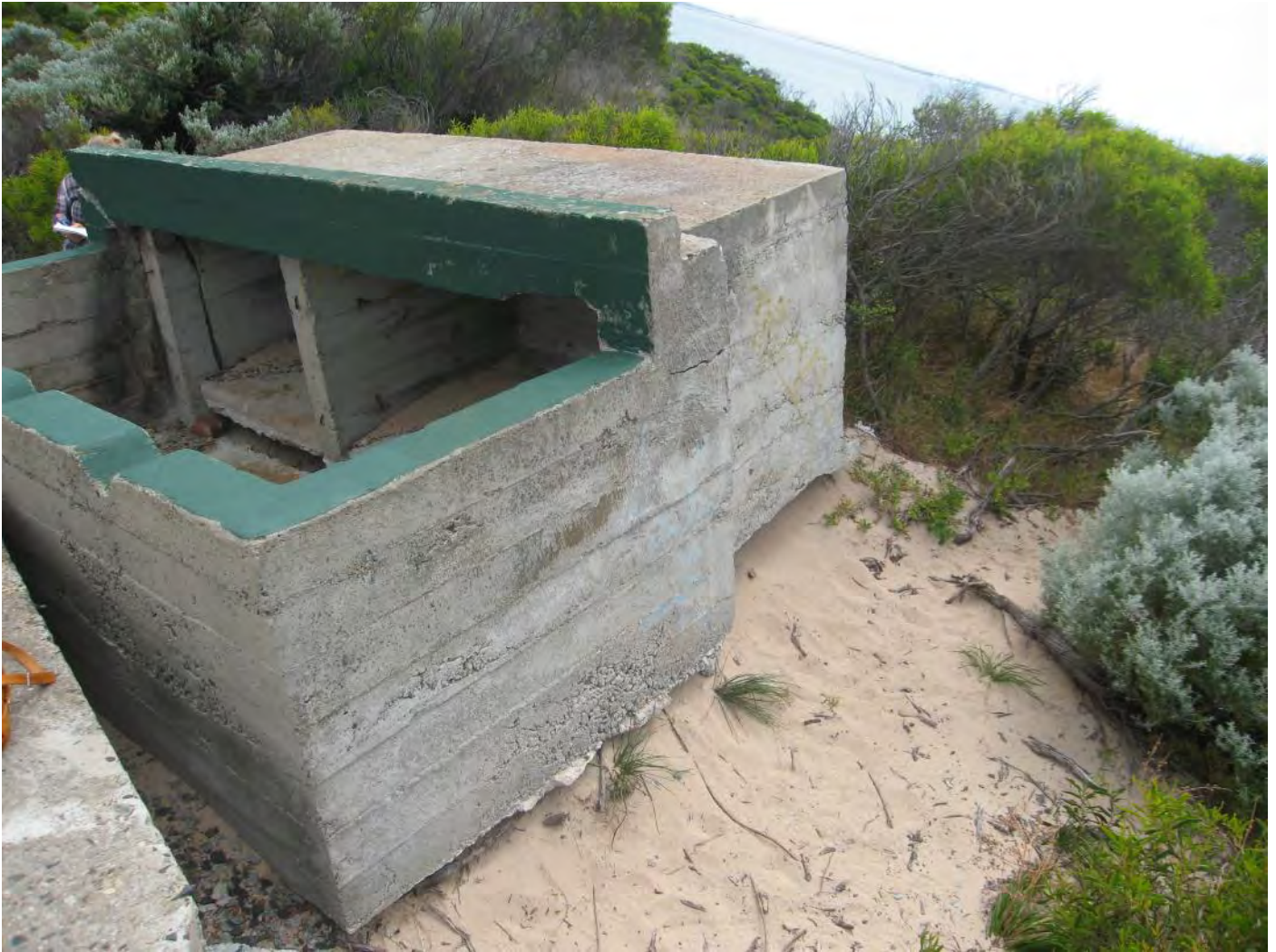
Figure 108: Gun Emplacement - Ammunition Store No. 1
