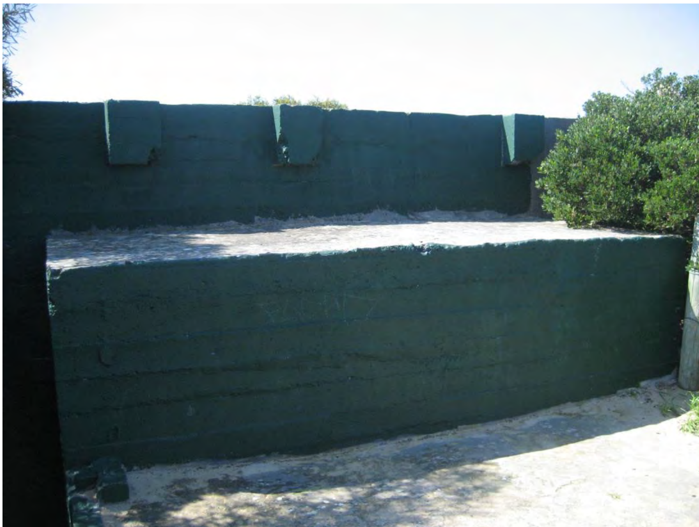
Figure 142: Ammunition Bunker No. 2 – south-west elevation
