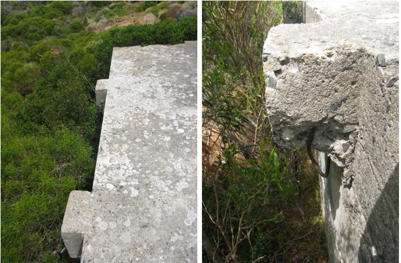
Figure 145: Ammunition Bunker No. 2 – Ventilation shafts
