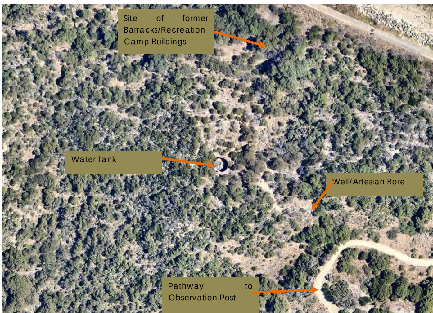
Figure 150: Water Tank Courtesy Nearmap, 2015
