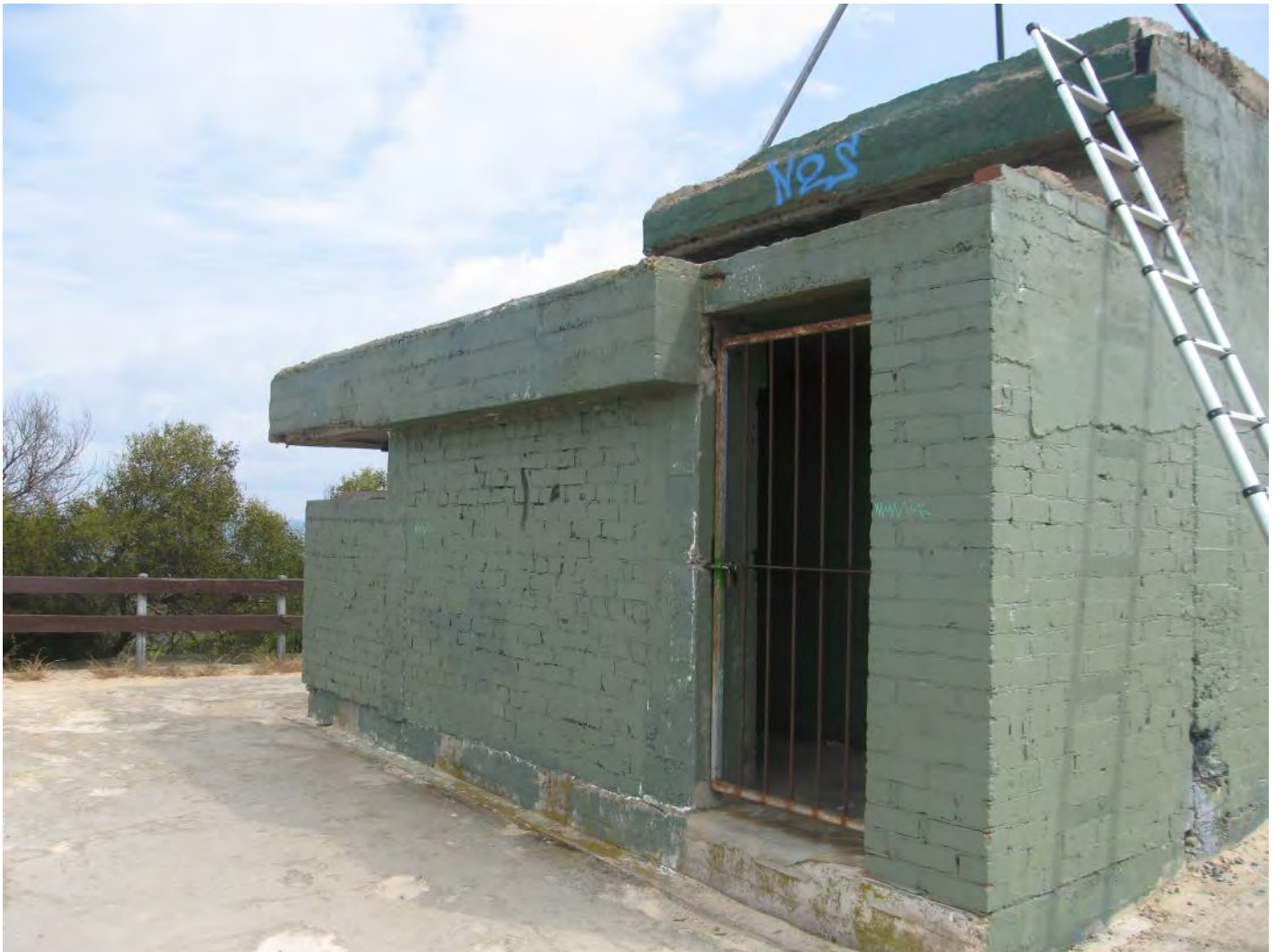
Figure 56: Observation Post – South Elevation
