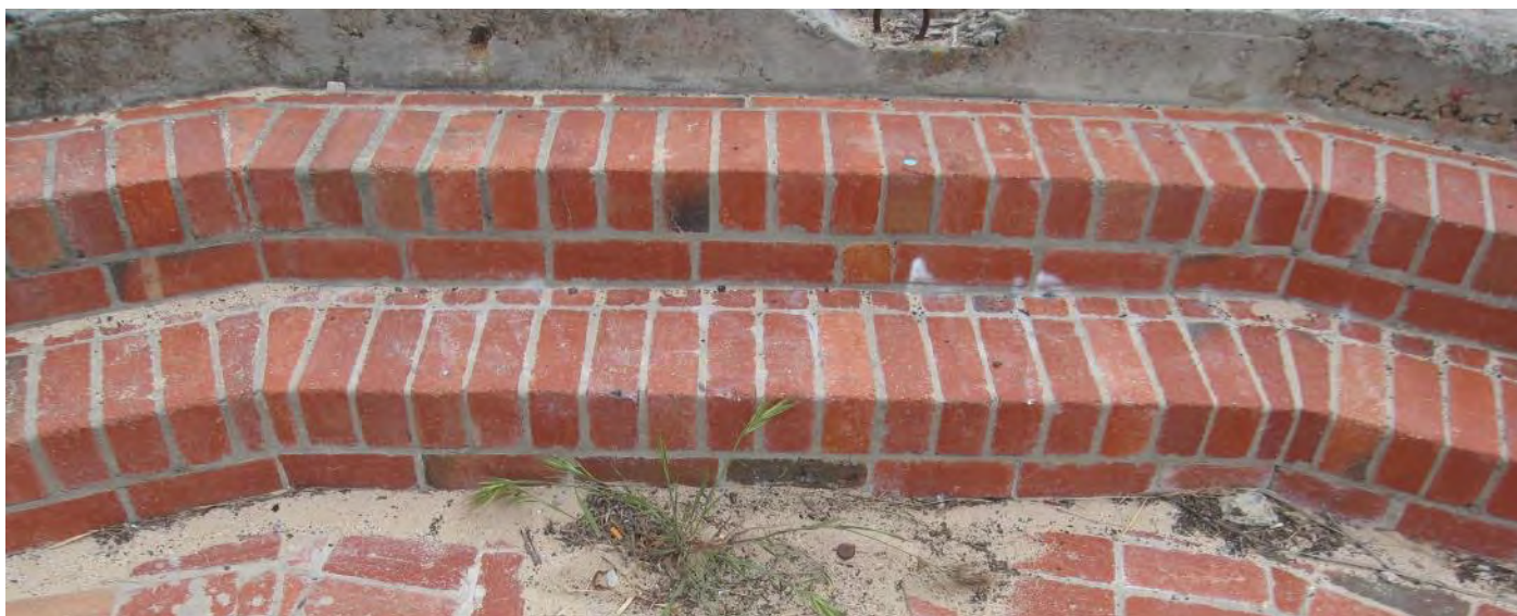
Figure 131: Gun Emplacement No. 2 – brick steps
