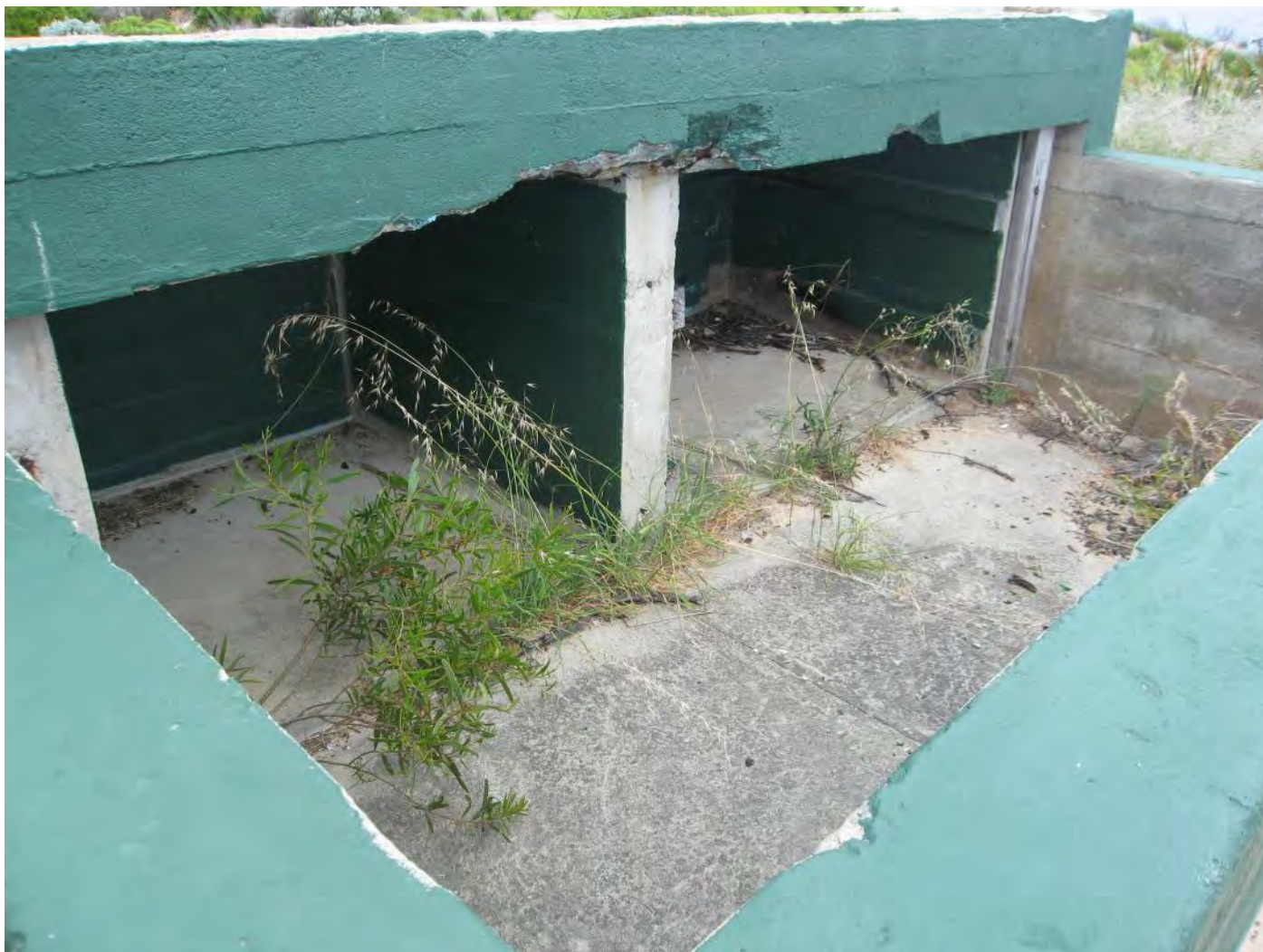
Figure 136: Gun Emplacement No. 2 – Ammunition Store 1
