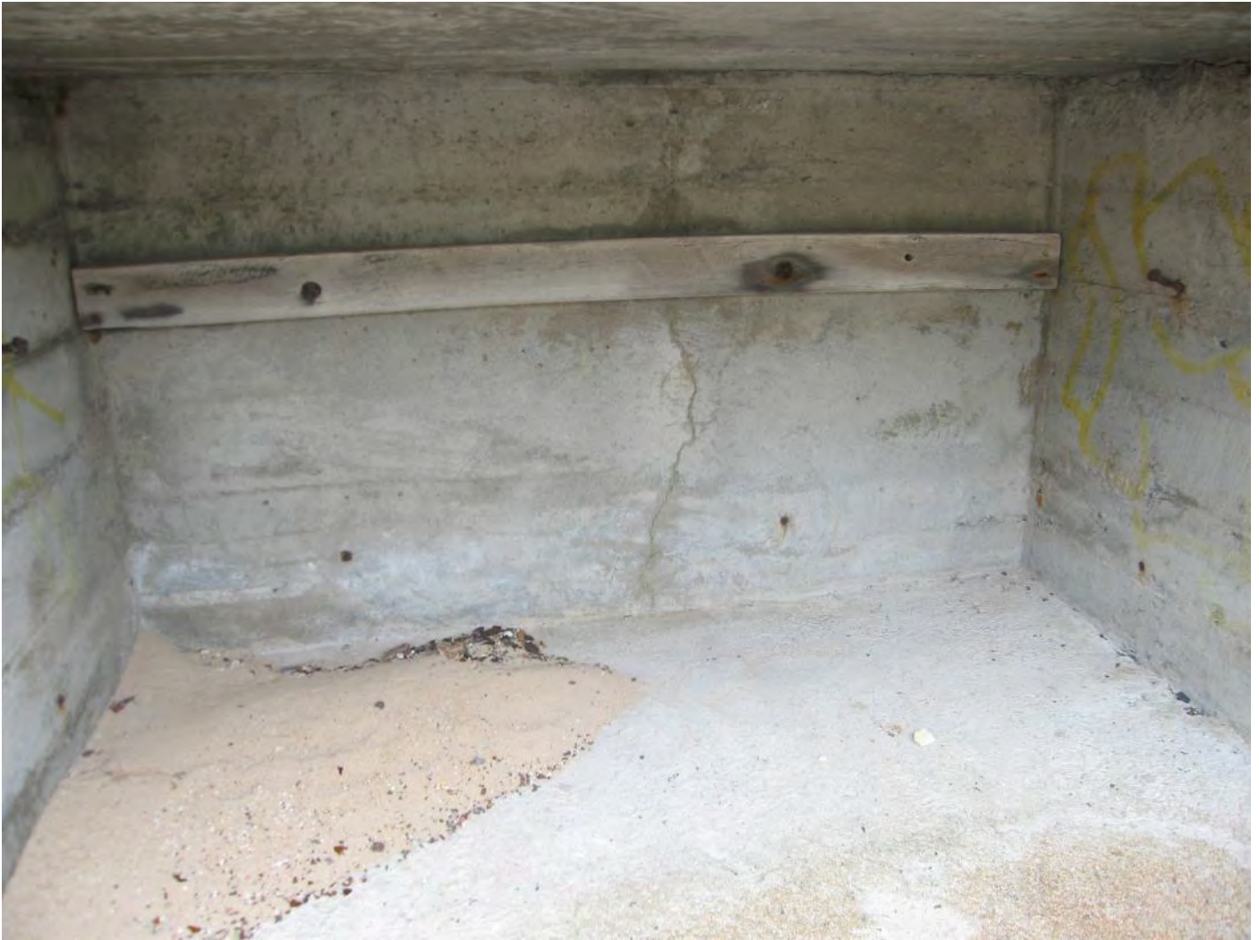
Figure 109: Gun Emplacement - Ammunition Store No. 1
