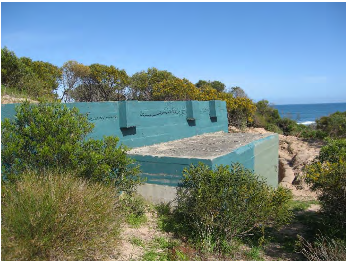
Figure 117: Ammunition Bunker – East elevation
