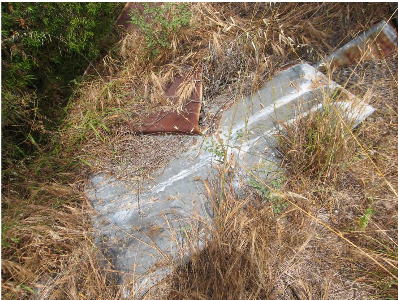
Figure 154: Water Tank – remnant roofing material
