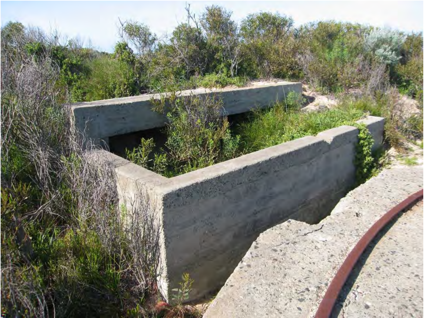
Figure 111: Gun Emplacement - Ammunition Store No. 2
