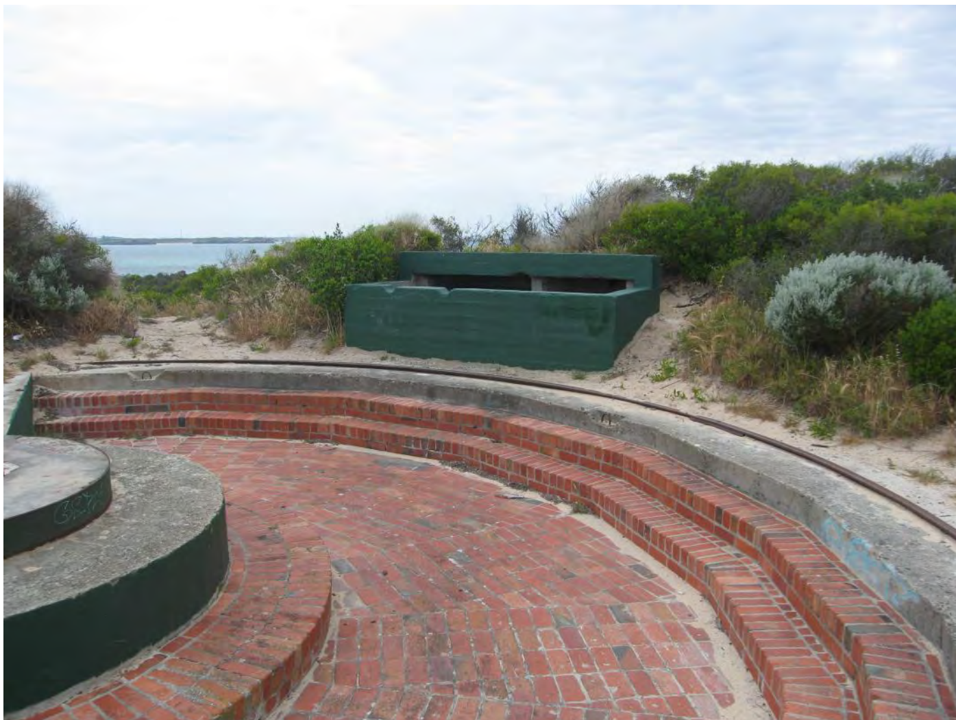
Figure 130: Gun Emplacement No. 2 – brick paving
