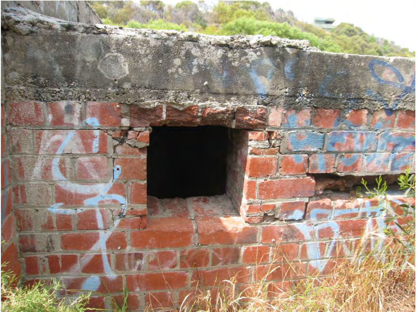
Figure 85: Operations Bunker – Openings in north wall
