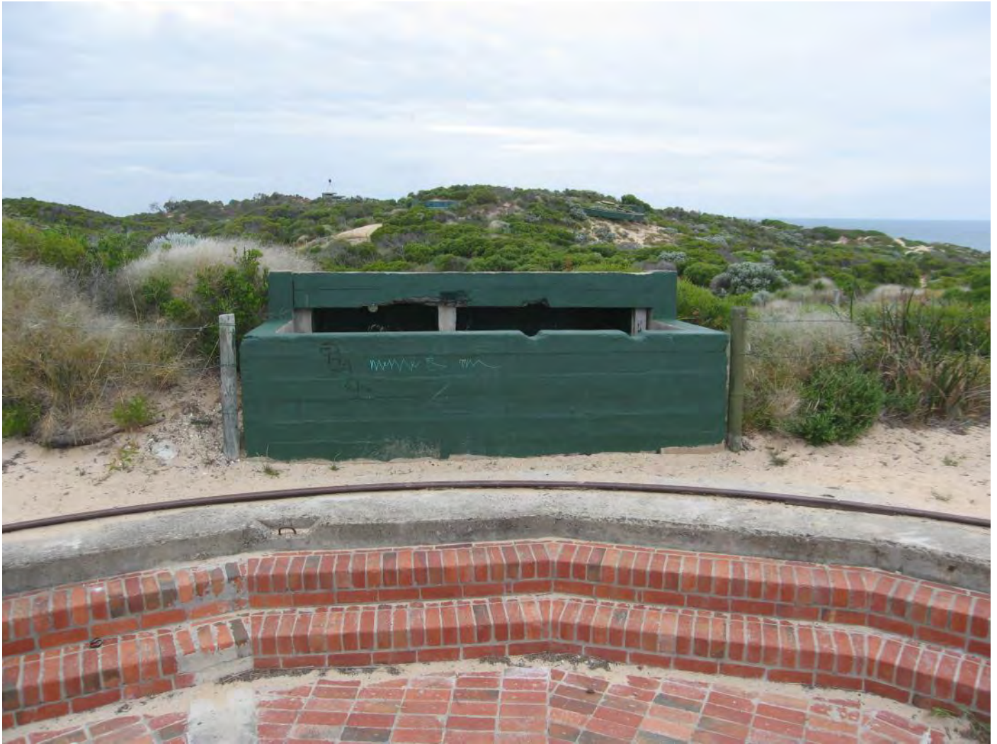
Figure 134: Gun Emplacement No. 2 – Ammunition Store 1
