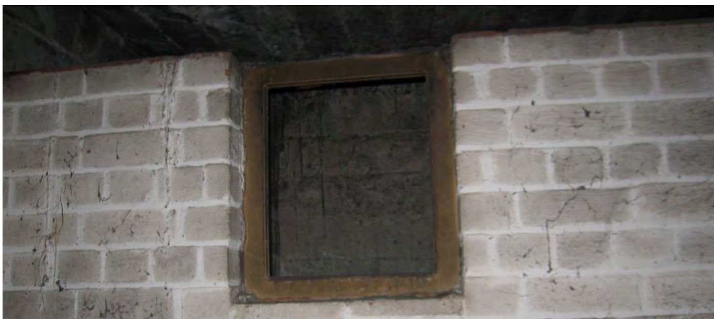
Figure 148: Ventilation openings in Room 2
