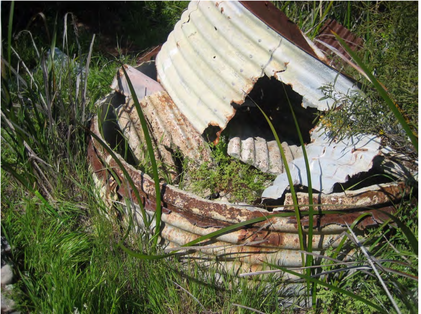
Figure 161: Former Well cladding
