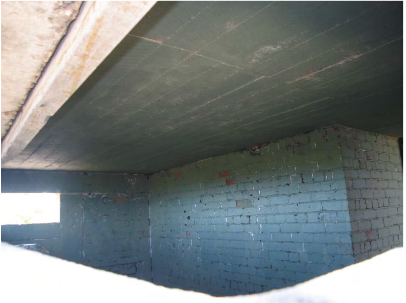
Figure 68: Concrete slab ceiling
