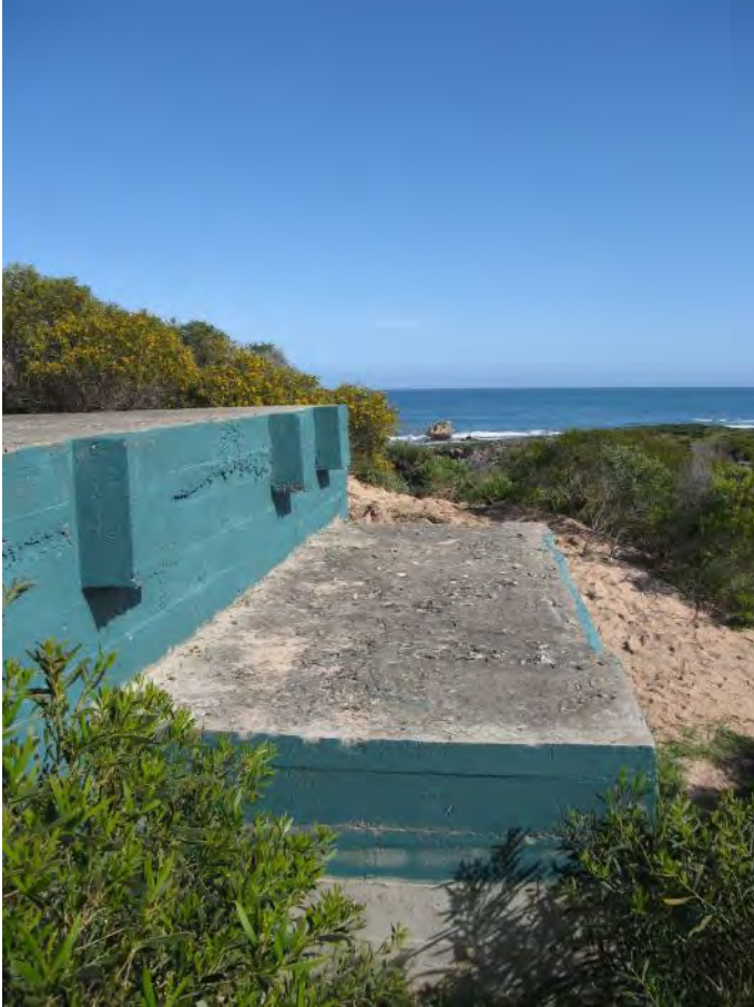
Figure 119: Ammunition Bunker – roof to entry tunnel
