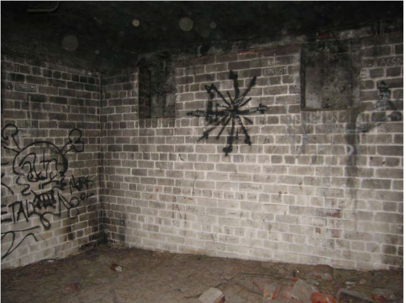
Figure 124: Ammunition Bunker – Room 2
