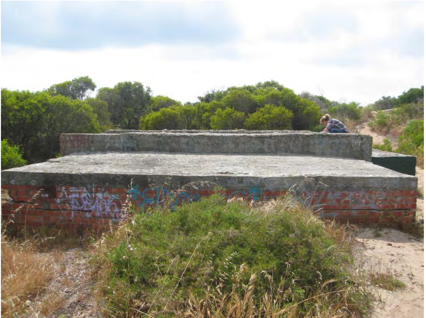
Figure 84: Operations Bunker – west elevation
