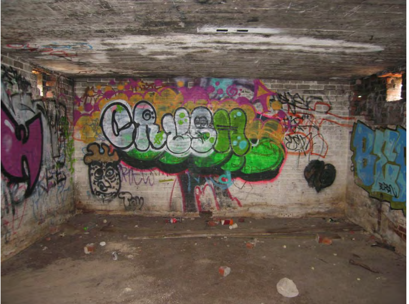
Figure 90: Operations Bunker – Interior (west wall)
