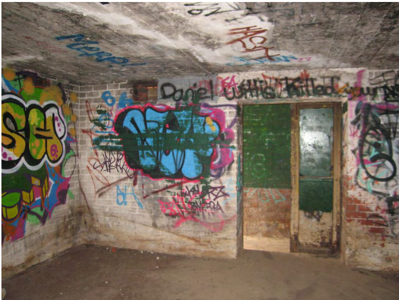
Figure 91: Operations Bunker – Interior (south wall)
