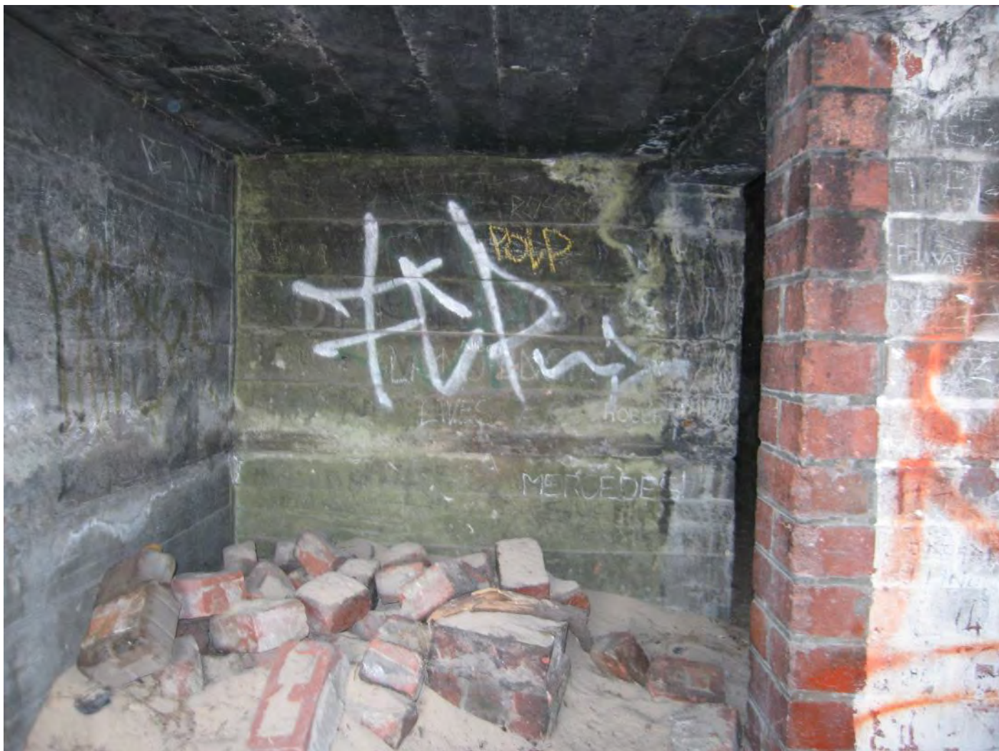
Figure 121: Ammunition Bunker – entry tunnel
