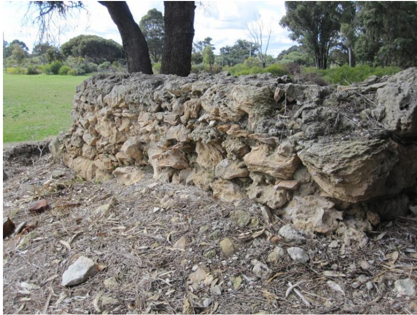
Figure 35 Eroding stonework
