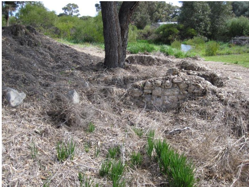
Figure 33 Debris infill and built up land levels
