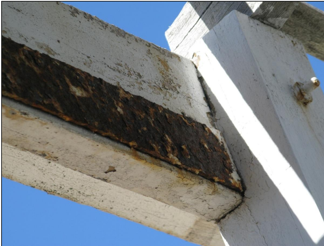
Steel plate to verandah beam on right side of house showing significant corrosion.
