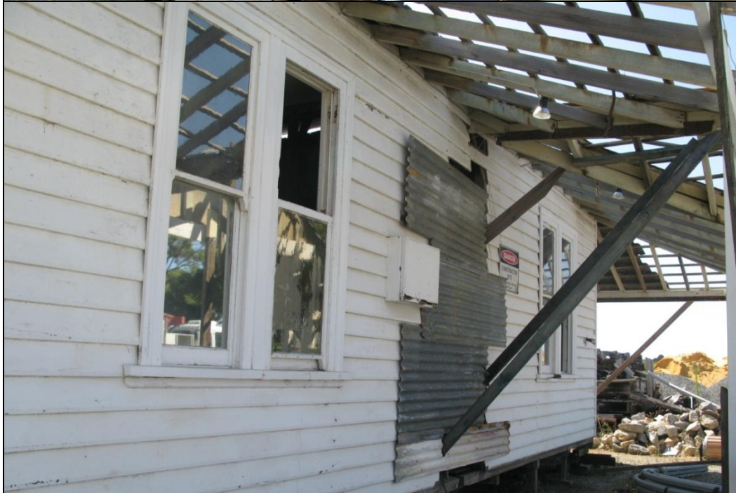
Front verandah showing paired double-hung sash windows.
