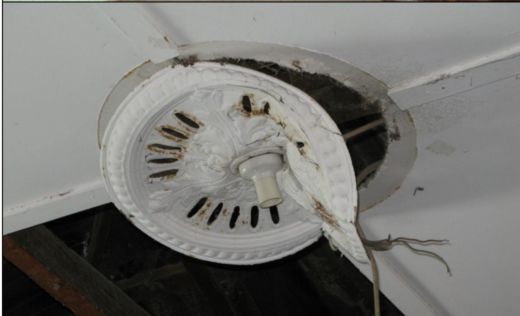
Damaged pressed metal ceiling rose to front left hand room. Battened plasterboard ceiling damaged.
