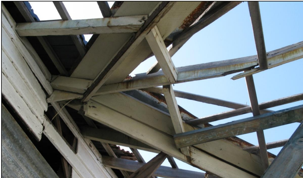
Damage to structure of projecting gable on front verandah
