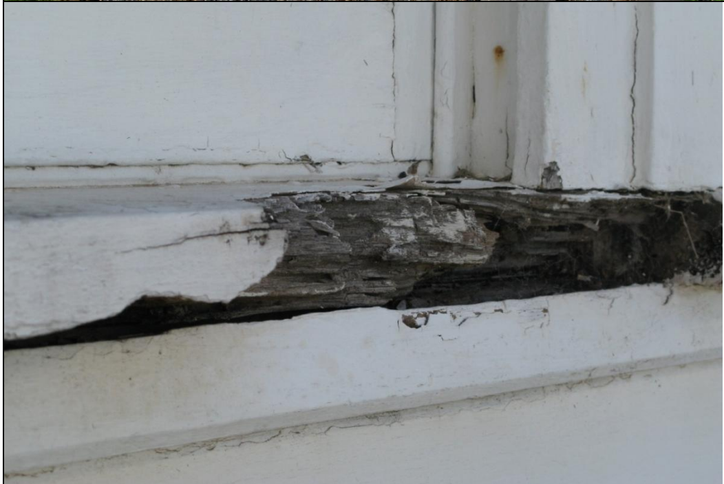
Advanced rot in timber window frame on front elevation.
