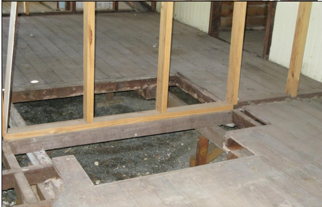
Hearth locations in right hand side front and rear rooms. Chimney removed for relocation of house.
