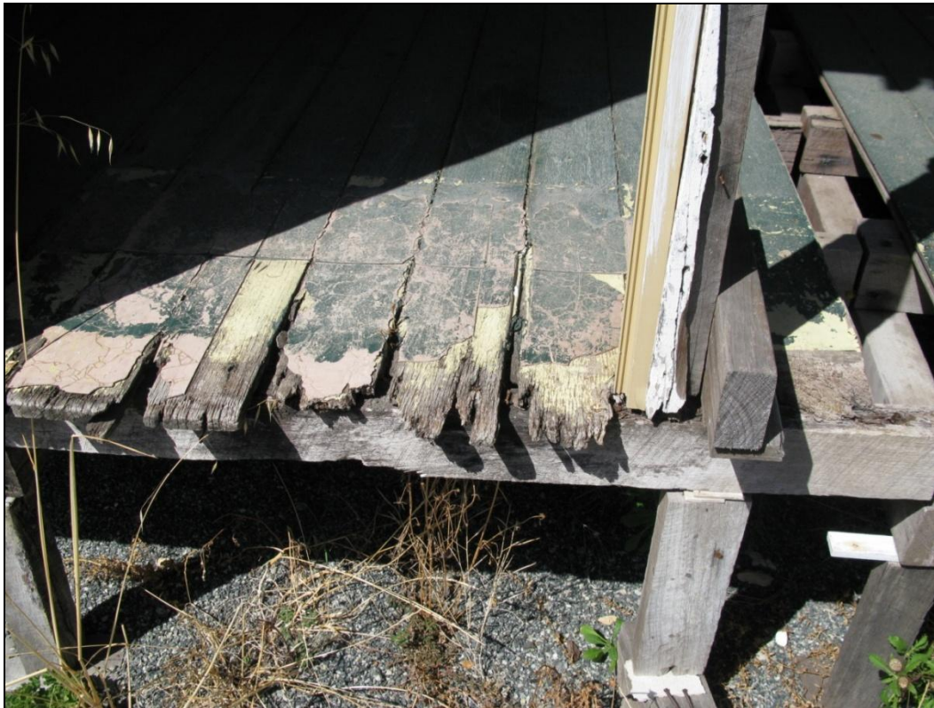
Significant weathering and rot to exposed floor-boards on back verandah (back door to kitchen area)
