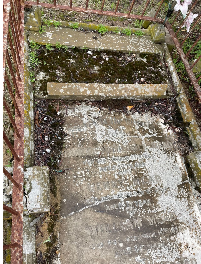
Figure 49 Cracked ledger stone (note this headstone moved from Fremantle Skinner Street Cemetery).
