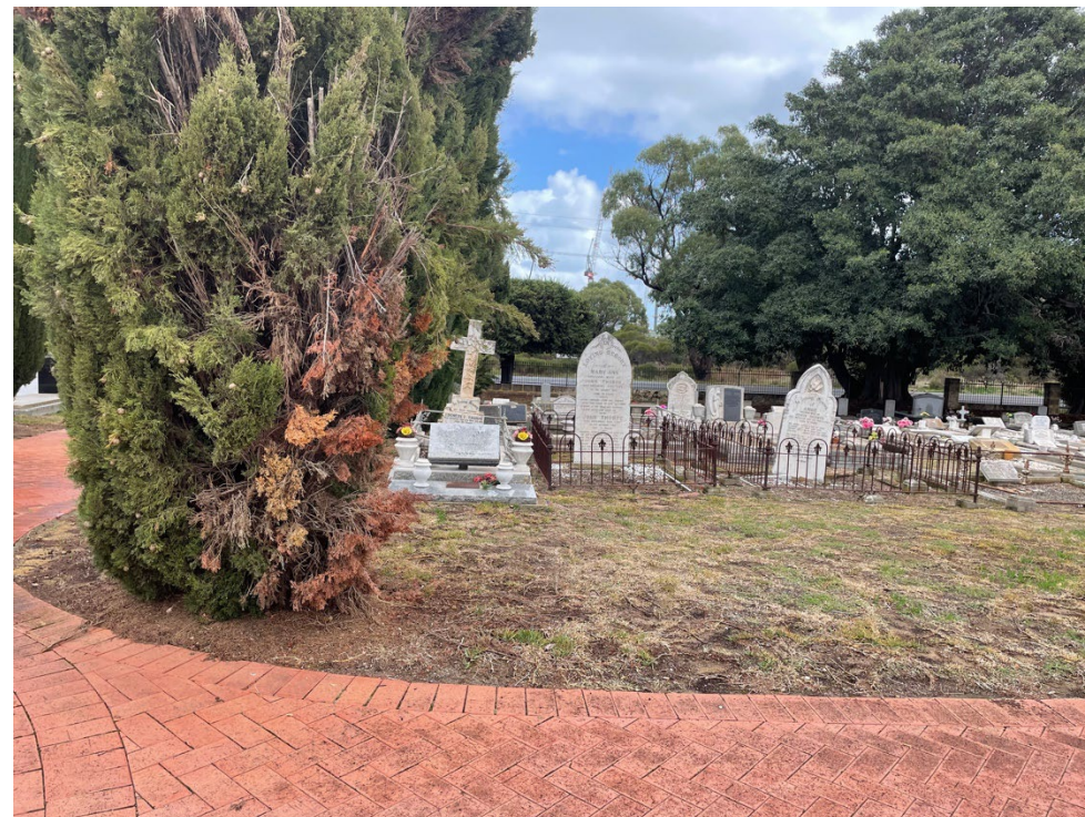
Figure 51 Graves suffering from subsidence adjacent to trees
