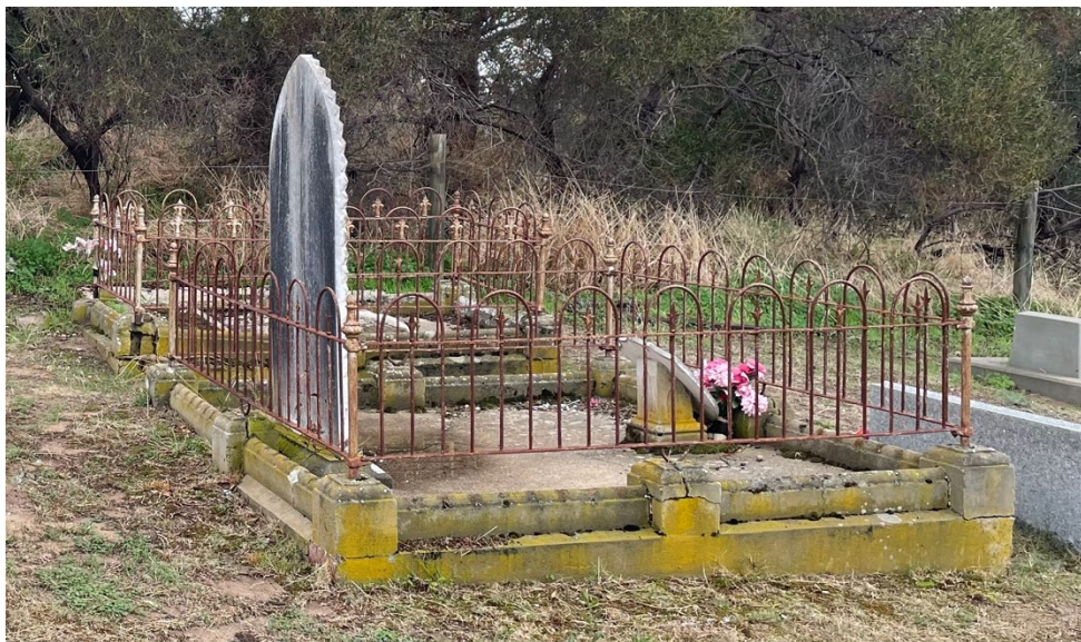
Figure 50 Cracked stone edging around the grave and rusted palisade fencing around the grave
