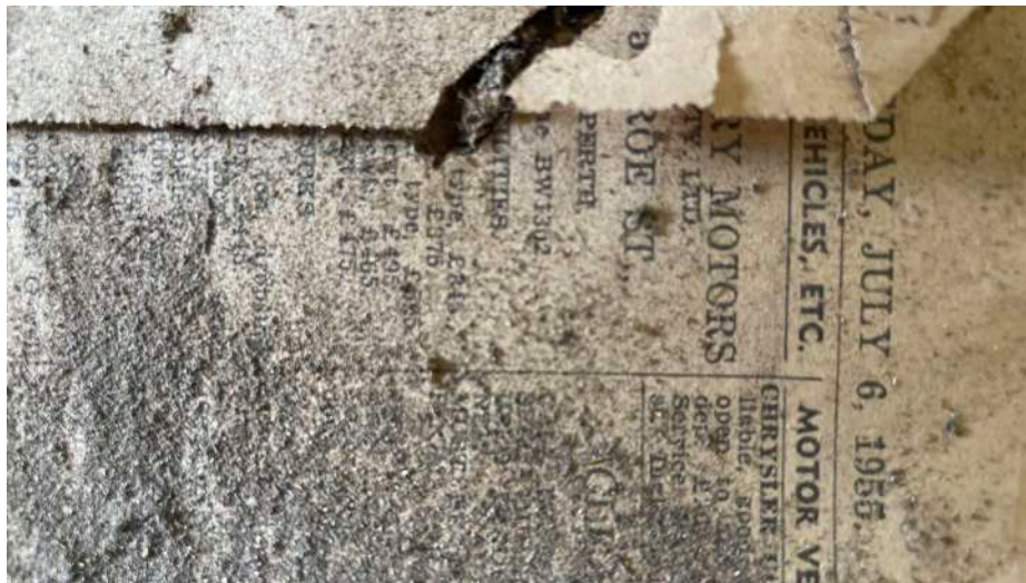
Figure 51. Newspaper lining below linoleum floor finish in Room 7 indicating rough date of installation (1955) (element, 2021)
