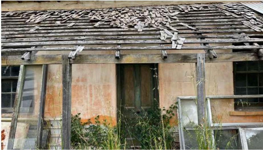
Figure 26. Front entry door to Day Cottage noting original shingles visible where corrugated sheeting has failed and ashlar lined external walls (element, 2021)
