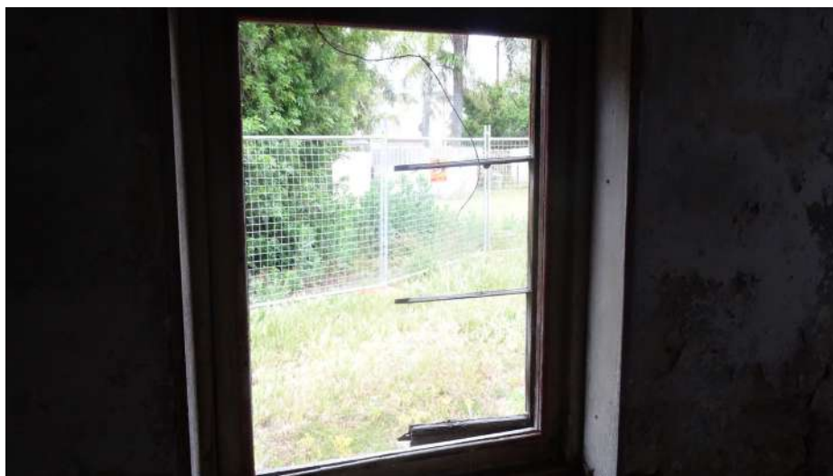
Figure 63. Northern window to detached kitchen noting missing timber joinery and glazing (element, 2021)
