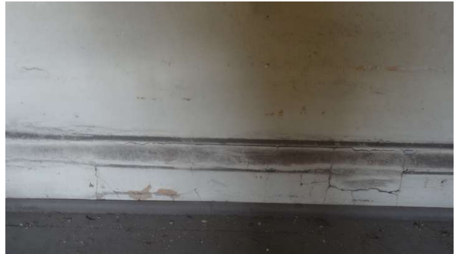
Figure 45. Plaster skirting noted throughout core rooms (element, 2021)
