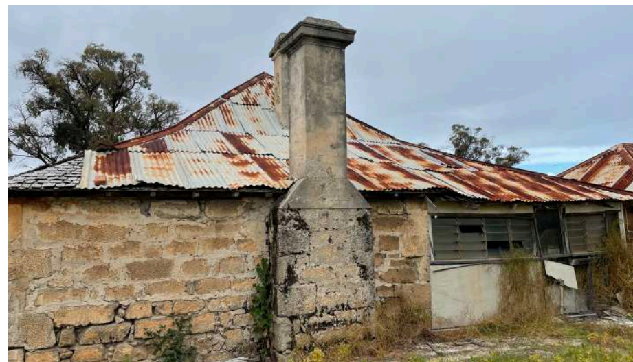
Figure 40. View to north facing facade noting external stone chimney structure and infill walls with glazed louvres to the north-west corner of the cottage (element, 2021)
