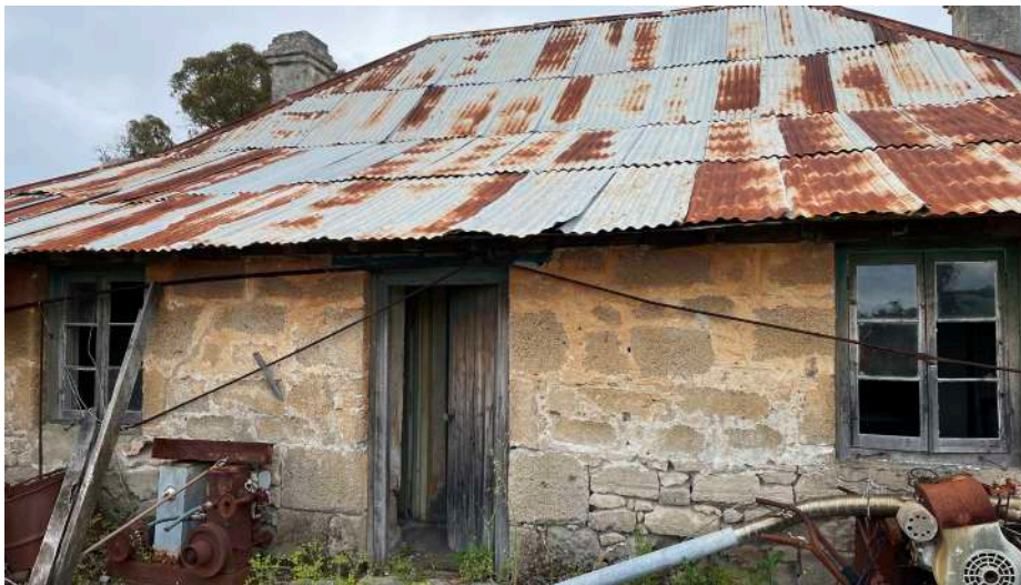
Figure 35. Rear facade (west facing) noting symmetry of window openings and chimneys in keeping with the front facade. External walls are uncoursed rubble stonework with no render or lining finish (element, 2021)
