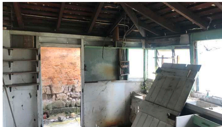
Figure 57. Room 2 looking west noting infill panelling, louvres and later fitout (element, 2021)
