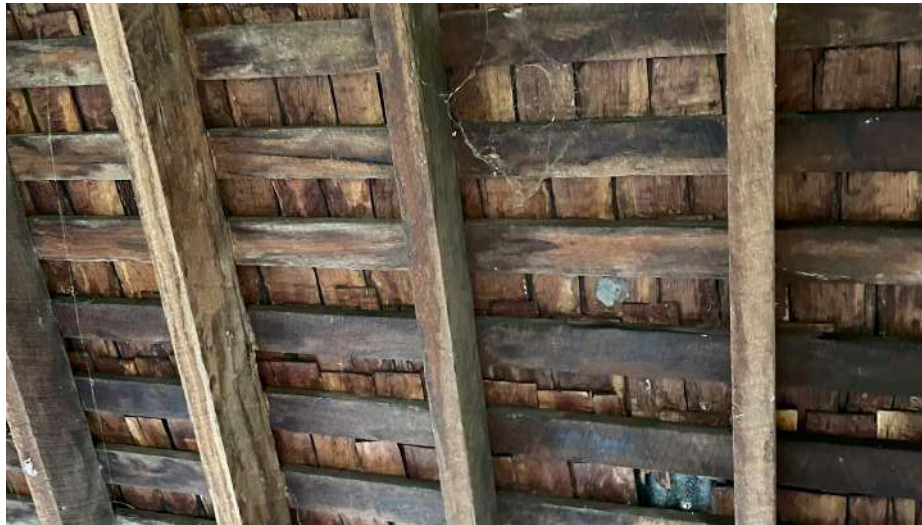
Figure 50. Rafters and underside of shingles exposed to all internal spaces other than the two core east facing rooms (element, 2021)
