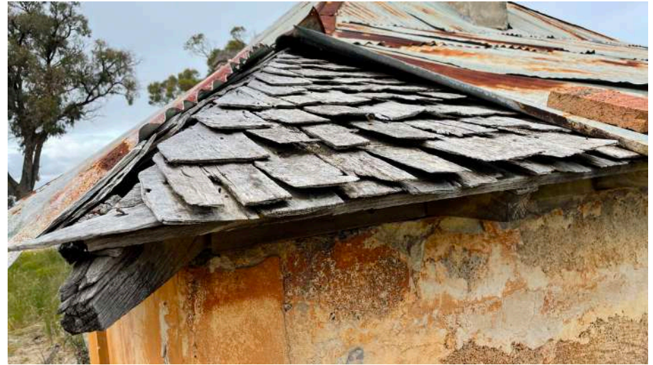
Figure 28. Detail of timber shingles to north-east corner where corrugated sheet covering has failed. Ashlar lined external wall finish visible below applied only to the front facade (element, 2021)
