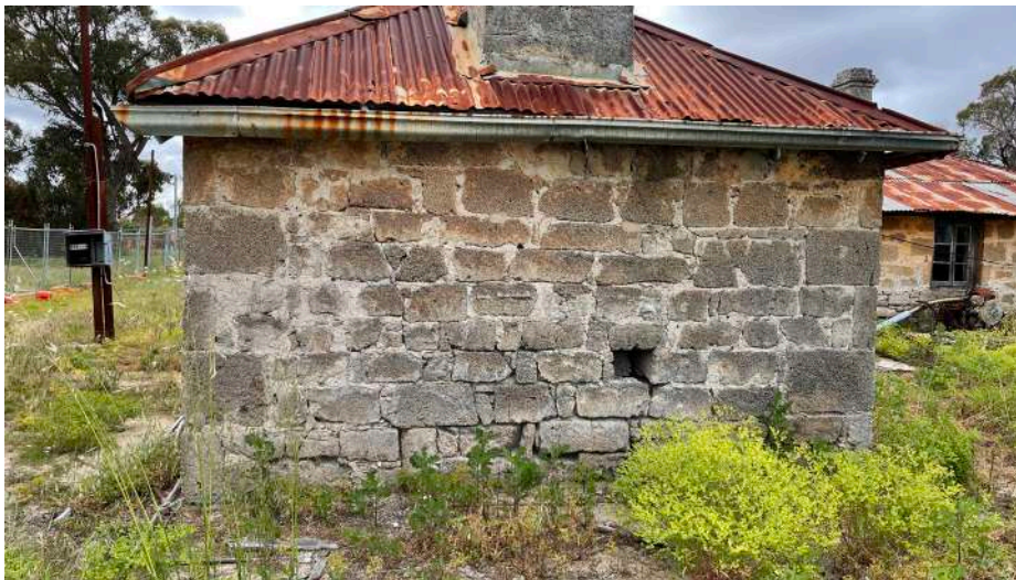
Figure 59. External view of detached kitchen looking east noting holes through stonework and cottage visible beyond (element, 2021)
