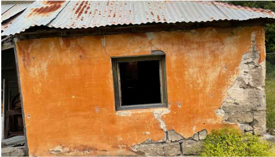
Figure 34. View of northern projecting room to front facade noting square window missing internal joinery. Ashlar lining finish is deteriorated to the northernmost corner, but otherwise visible. Orange pigmentation highly visible to this face (element, 2021)
