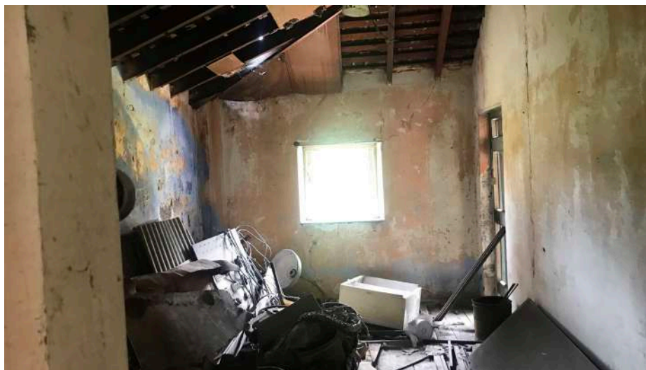
Figure 54. Room 3 looking east. Later ceiling linings have been nailed to the underside of rafters | (element, 2021)
