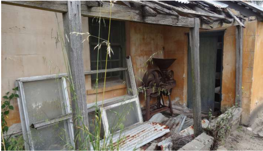
Figure 30. Front verandah noting low height stone wall, ashlar lining, double hung sash window to front facade and timber door to north eastern room (element, 2021)
