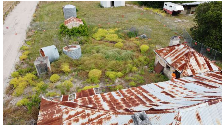
Figure 67. Aerial view to rear of the lot looking west noting exposed toilet structure, collapsed water tank and overgrown laundry structure beyond (element, 2021)
