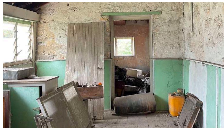
Figure 56. Room 2 looking east noting infill panelling, louvres and later fitout (element, 2021)
