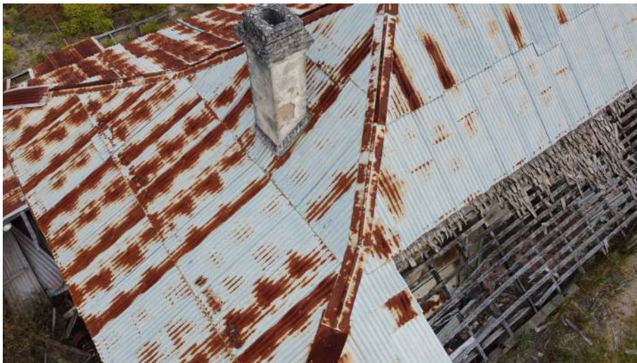
Figure 27. Aerial view from the south-east corner of Day Cottage noting corrugated sheet finish over timber shingles and stone chimney (element, 2021)
