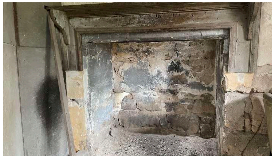
Figure 65. Fireplace to detached kitchen noting significant holes to low level stonework (element, 2021)
