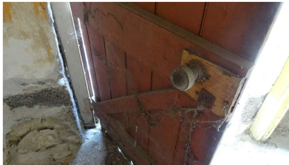
Figure 49. Rear ledged and braced timber entry door in Room 5 (element, 2021)
