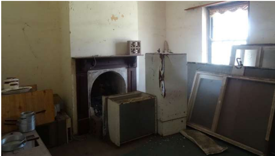
Figure 43. Room 6 noting fireplace, exposed timber floorboards, plaster ceilings and wall finishes with evidence of earlier schemes of decoration visible (element, 2021)
