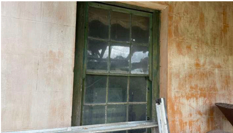
Figure 31. Detail of double hung sash window to front facade and ashlar lining finish with visible orange pigment (element, 2021)
