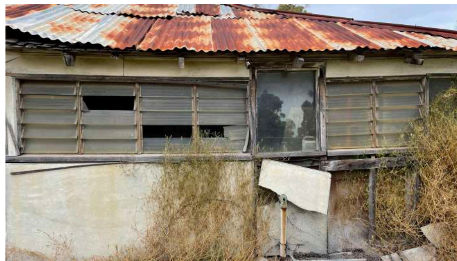
Figure 41. Infill walling to the north-west corner of the cottage noting extent of glazing to the upper half of the external walls (element, 2021)
