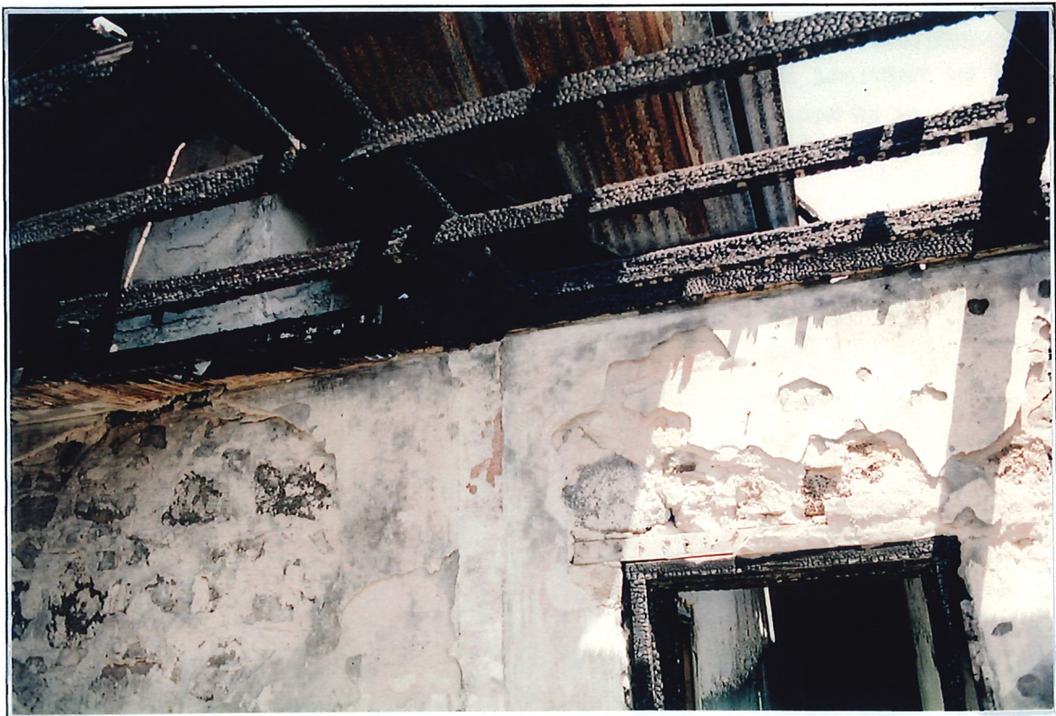
Figure 3.21 Portion of the south wall of the central front room. Diagonal grooves on the sides of the chimney (top LHS of photograph) are evidence of the alignment of an earlier roof which pitched off this wall. Vertical marks on the wall surface immediately to the left of the door are evidence of a stud wall which has been removed.
