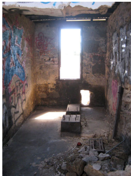
Photo 28 Internal view of Room B looking north, showing remains of concrete engine mounts in the center and boiler in the southern corner
