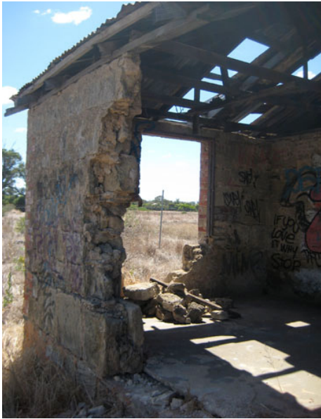
Photo 31 View showing collapsed walls in the northern corner
