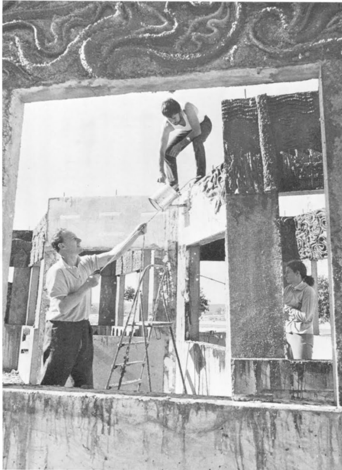
Early, crude Sculp-crete techniques operated by Ralph Hibble (top), Erica Ritter and Paul Ritter, on the V-shaped units in the casting yard. The various types of friezes can be identified.
