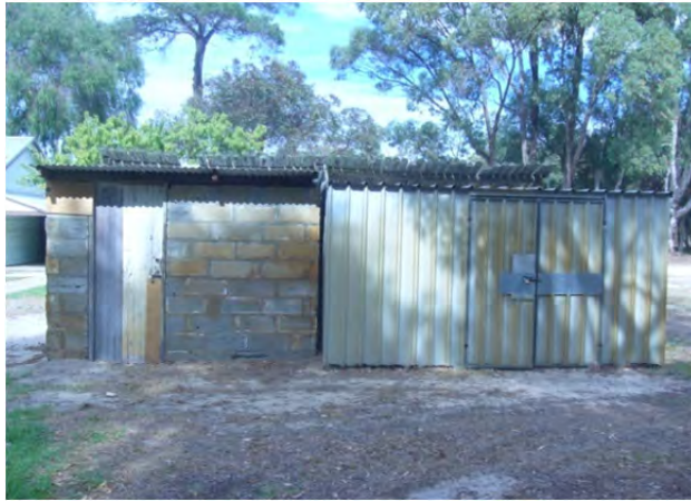
Figure 86. Bldg 4 Cement besser block store with corrugated iron addition (replaced in 2011), north elevation.
