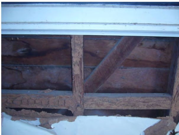
Figure 74. Bldg 2 main room white ant damage.
