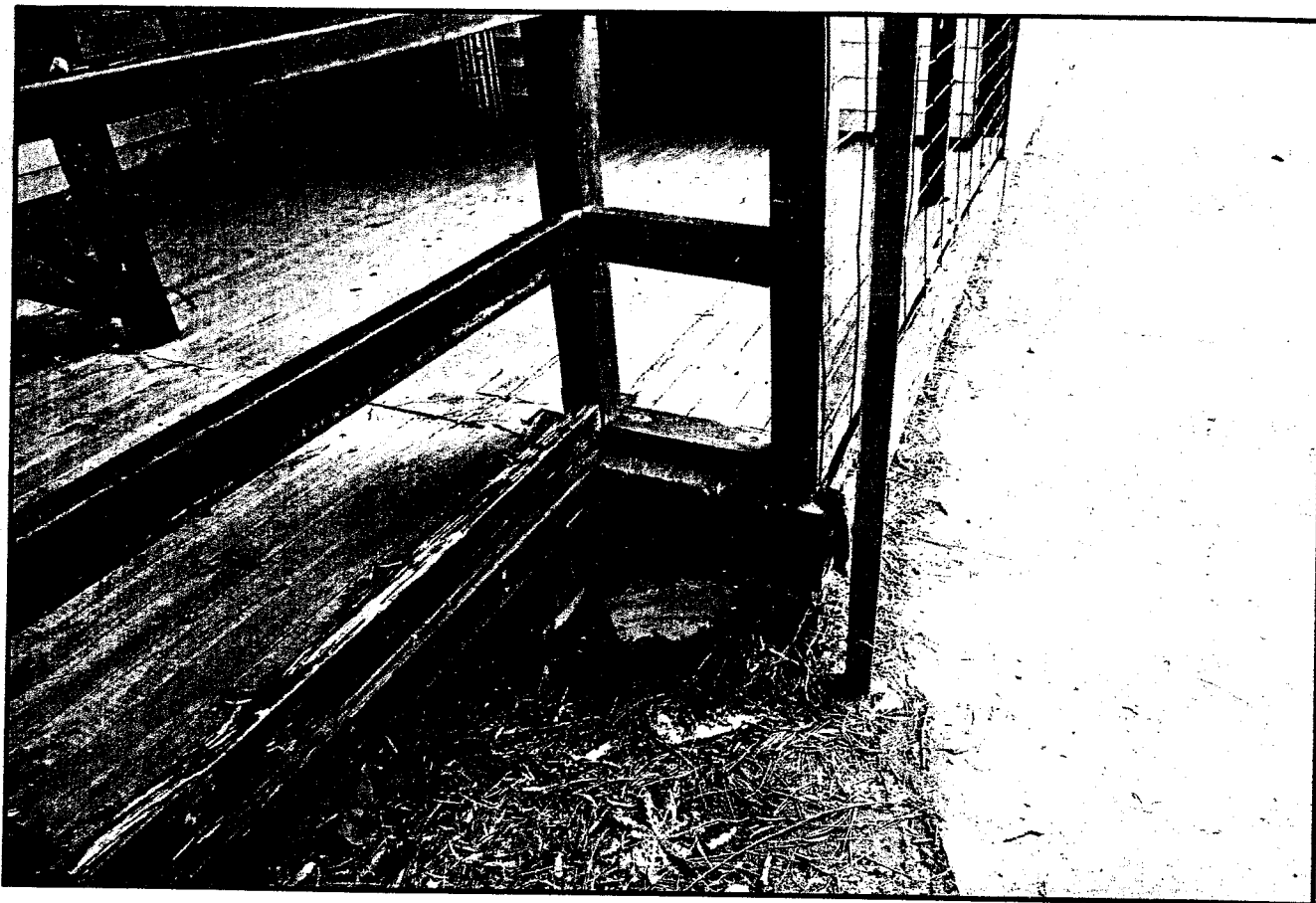
Photo 7 - Front deck has suffered from wood rot and members require replacement
