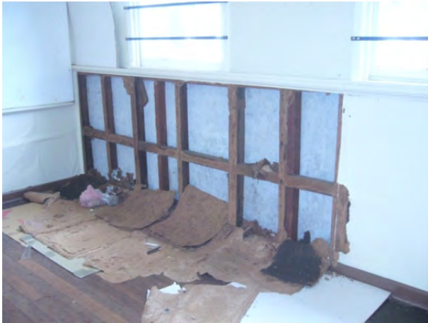
Figure 72. Bldg 2 main room white ant damage.
