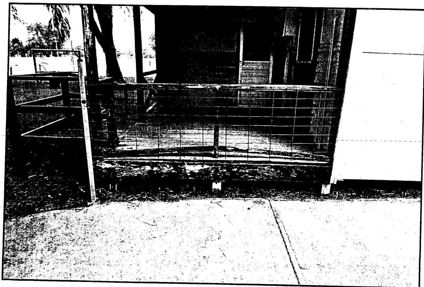
Photo 8 - Front deck has suffered from wood rot and members require replacement
