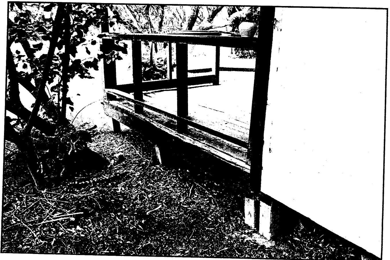
Photo 6 - Note rotation of stumps (typical)
