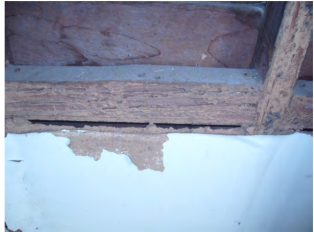
Figure 73. Bldg 2 main room white ant damage.
