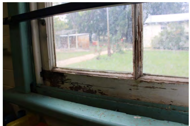
Figure 42. Bldg 1 main room window damage, north wall.
