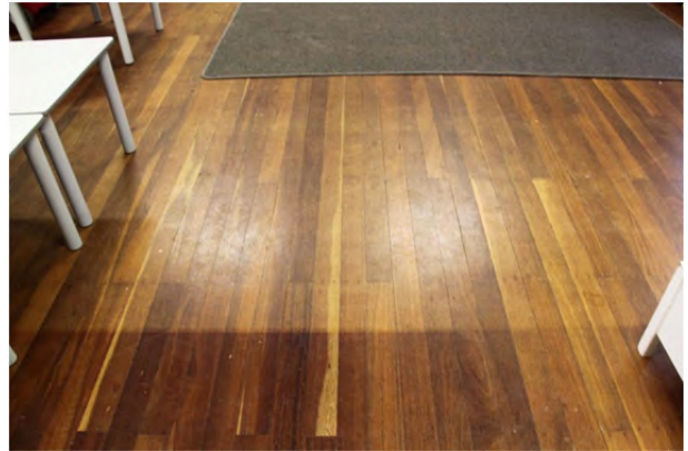
Figure 40. Bldg 1 floorboards replaced in main room
