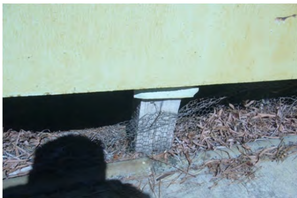
Figure 29. Bldg 1 north elevation timber stump.
