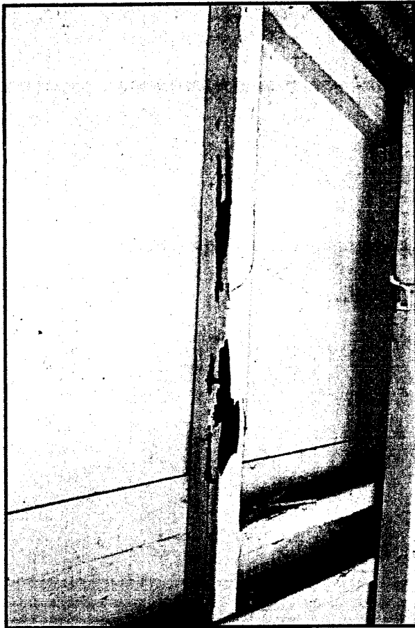
Photo 13 - Termite damage to porch wall stud
