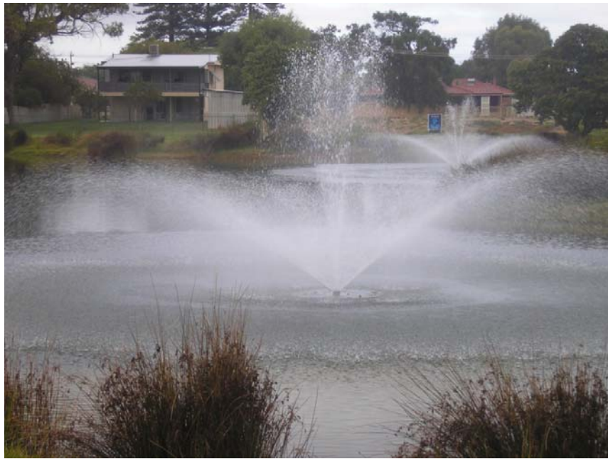
Plate 2: Rotary Park showing surface aerators.
