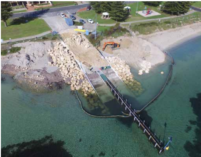
6.2 Rock Armour at Palm Beach boat ramp
